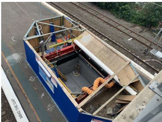
Excavation and piling work for the new platform lift and construction of the Dangar Road lift continued in February.
