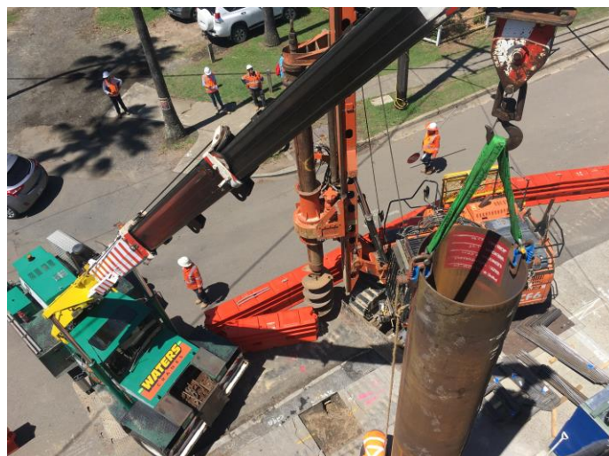
Excavation and piling work for the new platform lift and construction of the Dangar Road lift continued in February.
