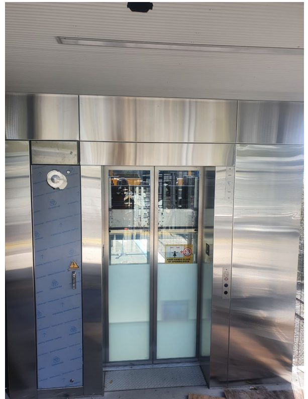
Image: Work on the two new station lifts is progressing well.
