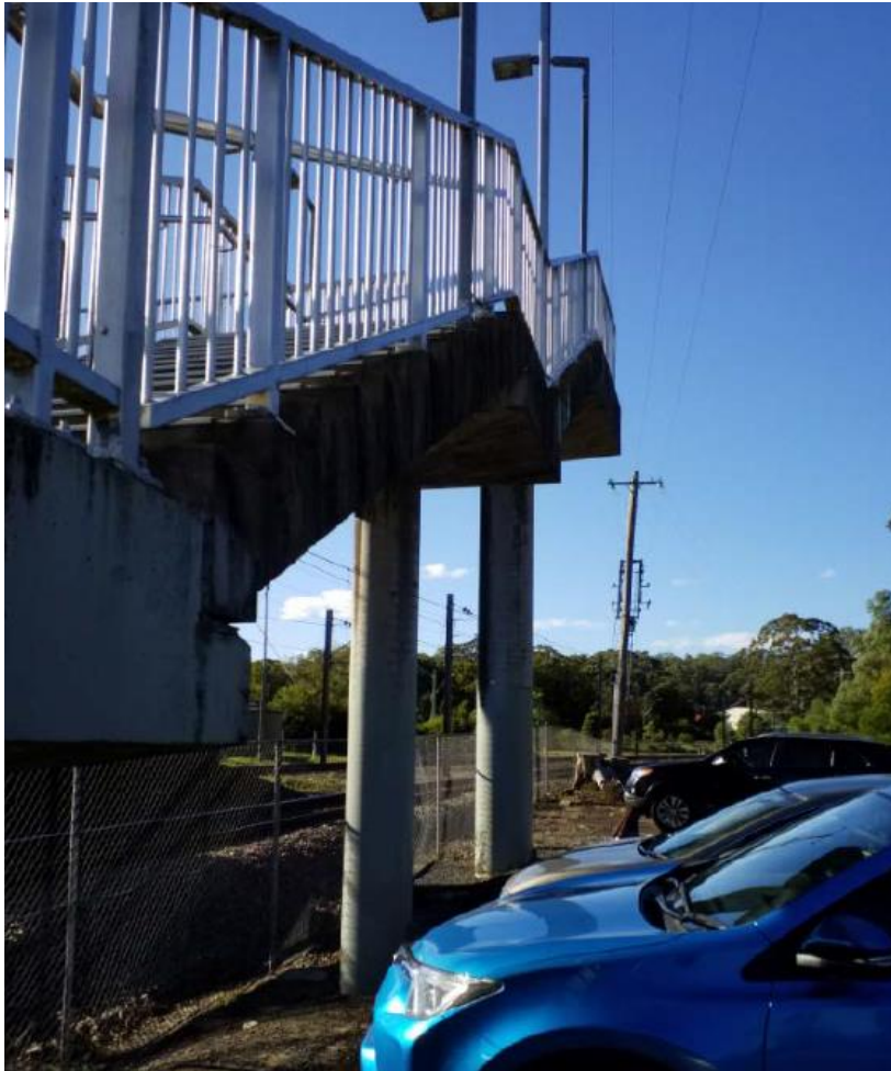
Figure 3-7 high voltage electricity lines cross the proposed Lift 3 location and would need to be realigned.
