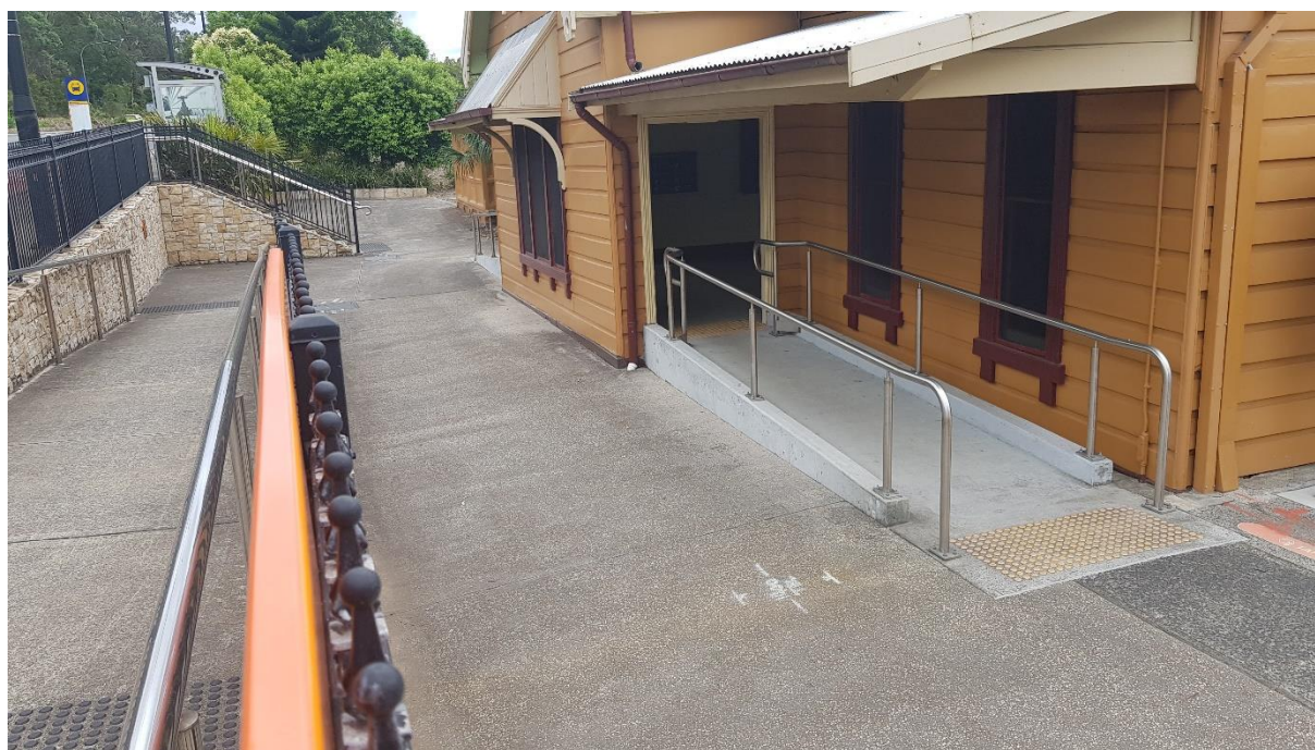
Figure 3-4 Existing non-compliant ramp to the timber station building on Platform 2
