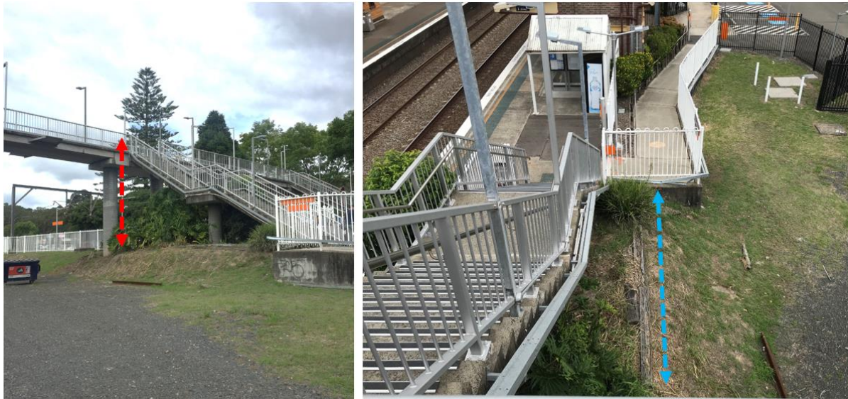
Figure 3-2 Location of lift servicing Platform 1 indicated by the dashed red line. The need for a retaining wall and a path to link to Platform 1 (dashed blue line) is evident in the image.
