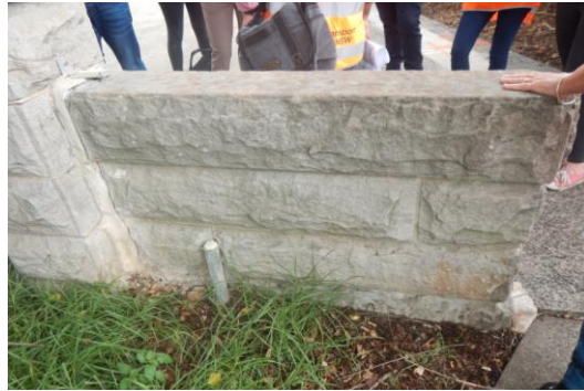
Figure 4-35: View of the dwarf stone wall and intrusive cement sand mix mortar.
