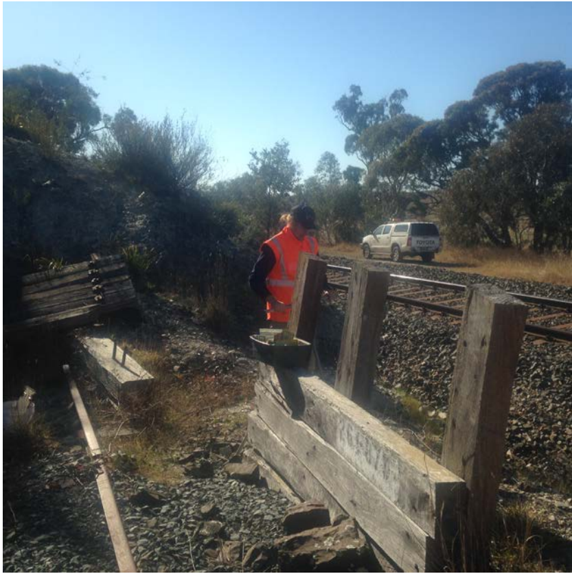
Baulk at the end of the Woodlawn Siding
