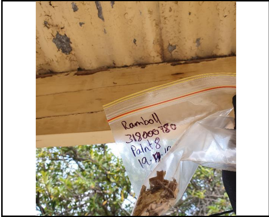
Photo 13: Station Masters Cottage external paint sample (PAINT8). Taken 19/12/19.
