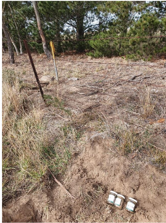
Figure 2.4.1 – Test pit with identified service in background.
