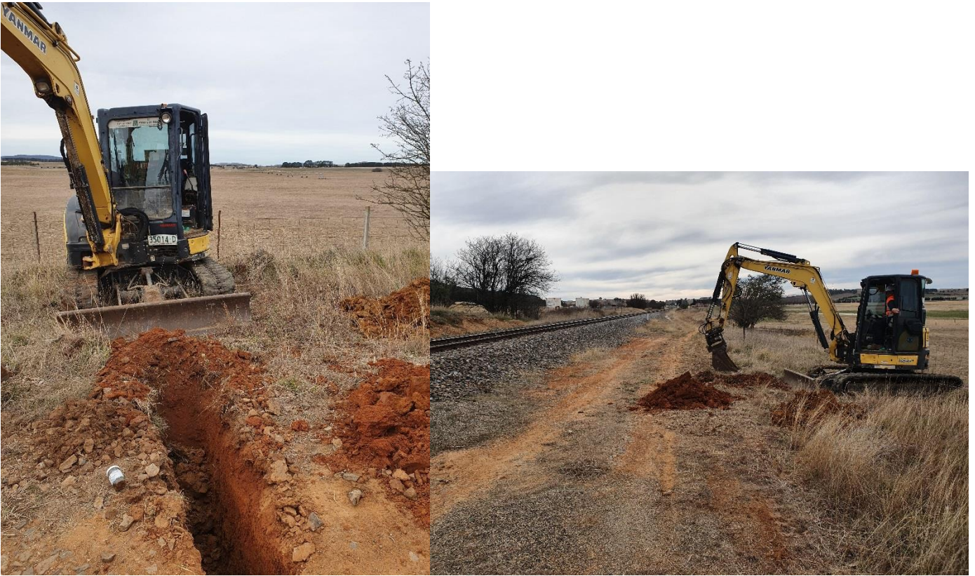
Figures 2.2.7 to 2.2.10 – Test pit location.
