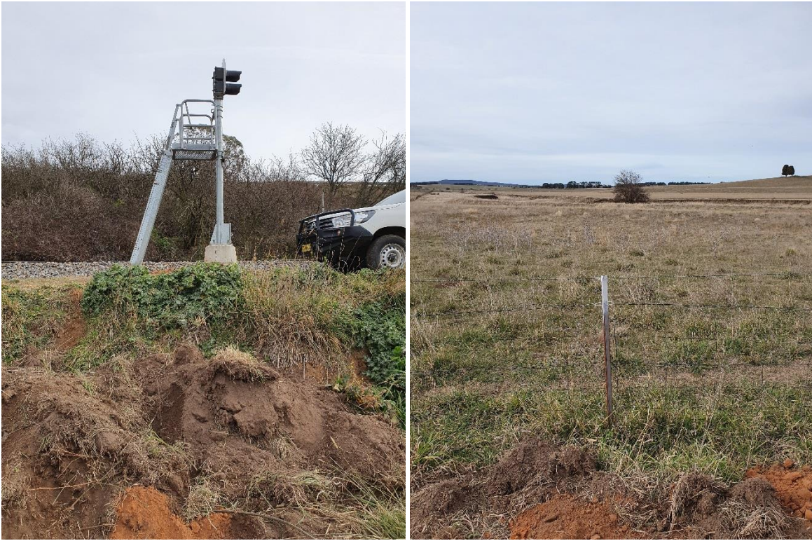
Figures 2.3.1 to 2.3.6 – Test pit location
