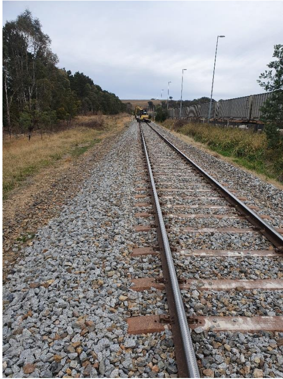
Figures 2.4.2 to 2.4.4 – Test pit location.
