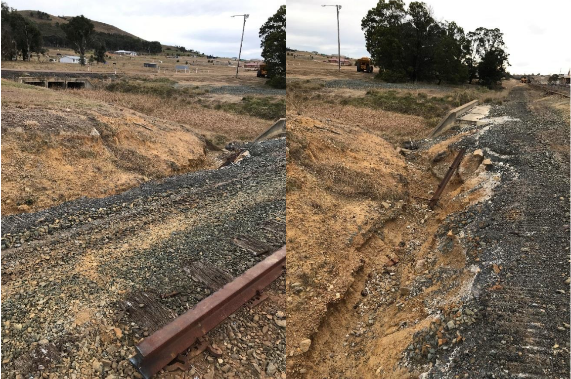
Drainage lines next to the culvert
