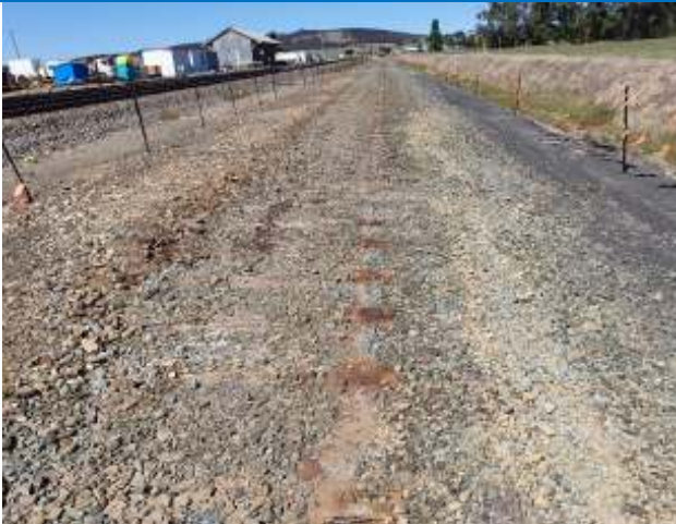
Photo 1: Track Adjacent Work Site.
