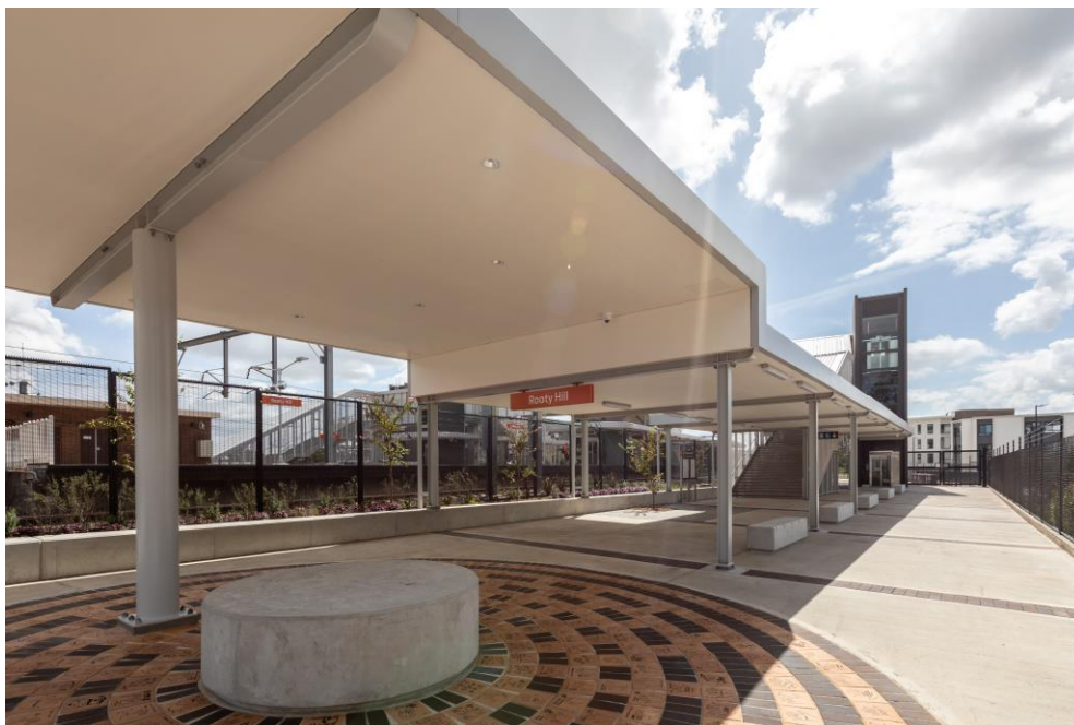
The 'Pride of Place' pavers in the Beames Avenue forecourt
