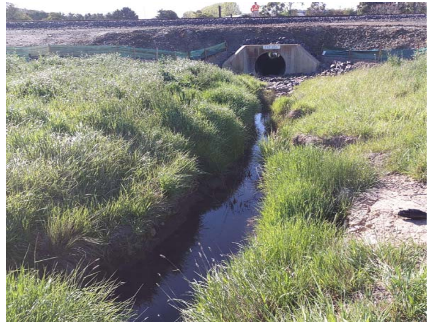
Culvert underneath rail line opposite Boyd Street
