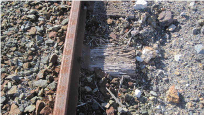
Figure 2: Siding Timber Sleepers
