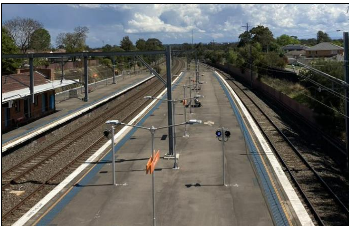
Photo 4.3 Views to the west along Platforms 1 and 2 taken from the footbridge
