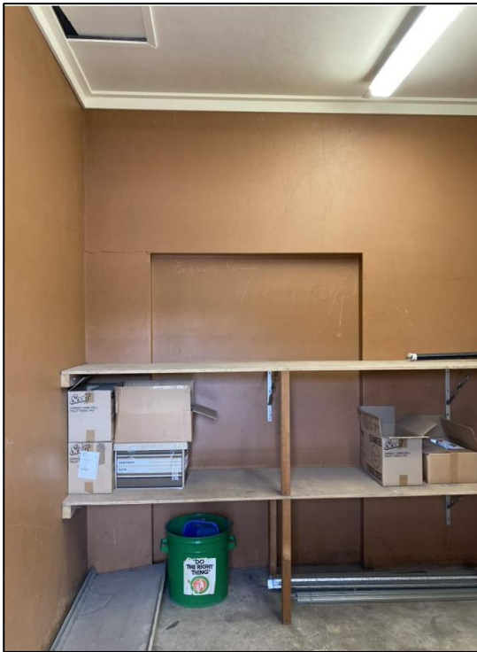
Photo 4.16 Station Building A, Storeroom
