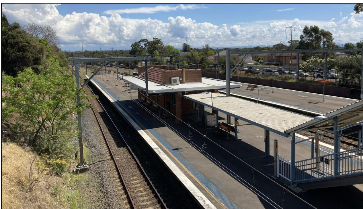
Photo 4.5 Views to Platforms 3 and 4 and Station Building A looking east from the Footbridge
