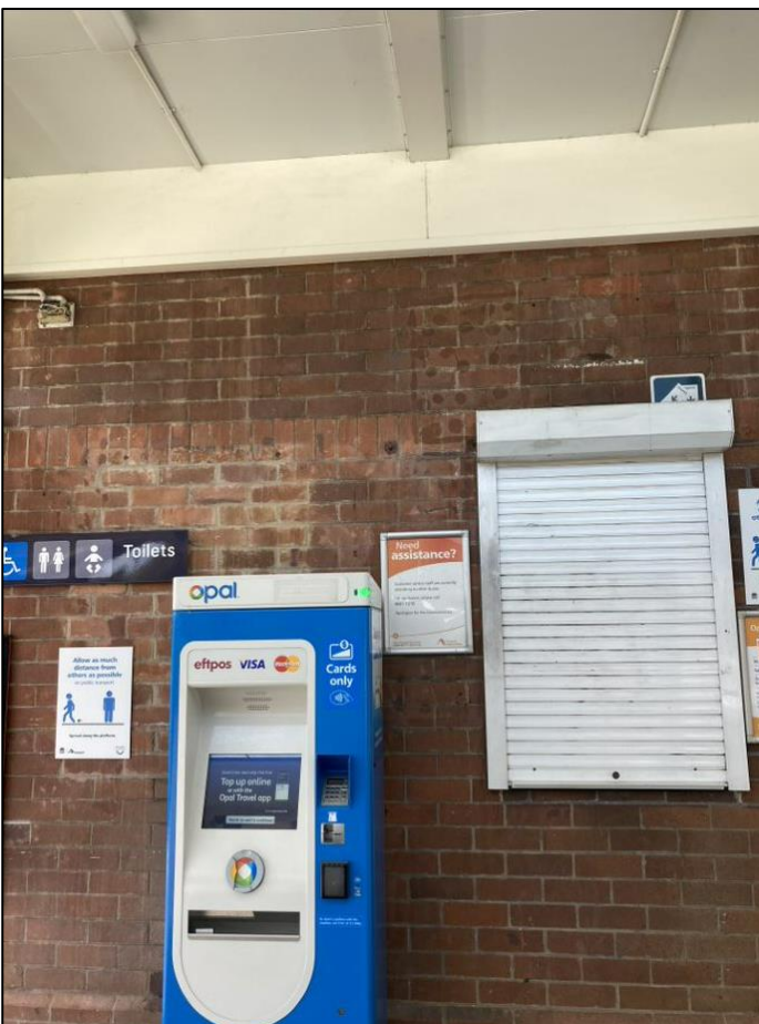
Photo 4.9 Station Building C, West Elevation
