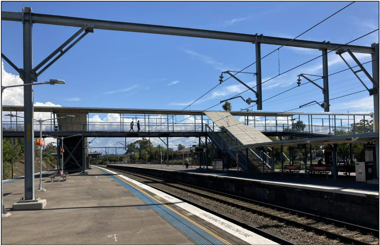
Photo 4.21 Footbridge, spanning over the platforms
