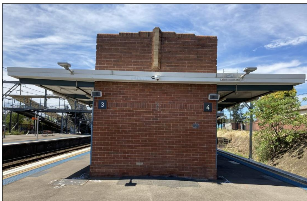
Photo 4.13 West elevation of Station Building A
