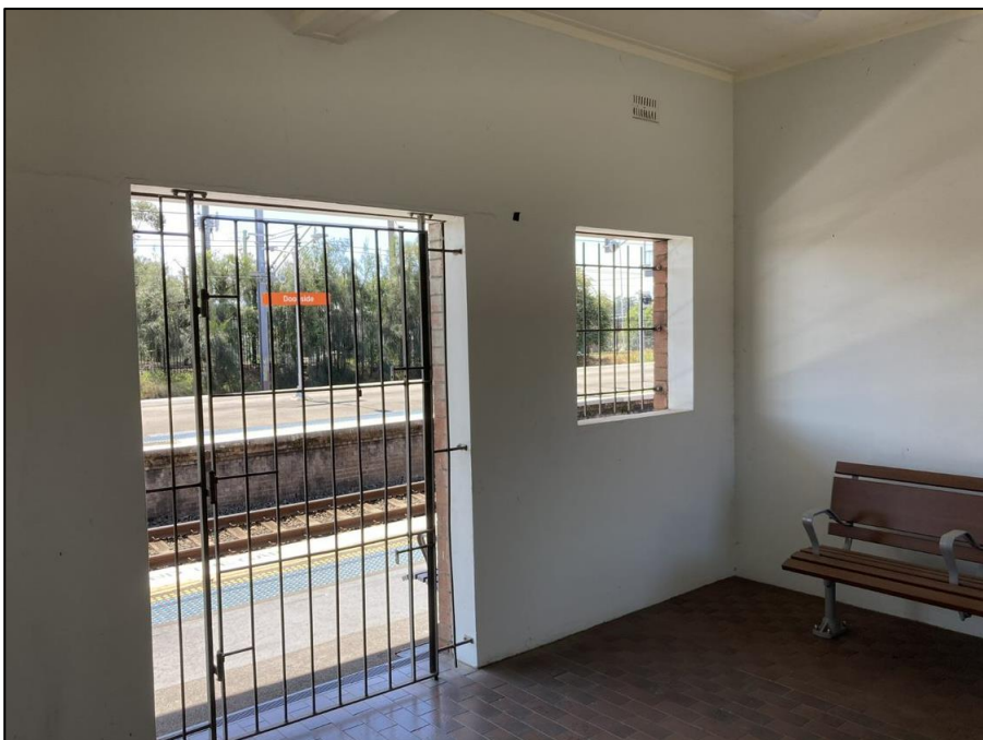
Photo 4.17 Station Building A, former waiting room in the central space
