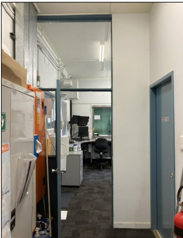
Photo 4.11 Partition wall and internal bathroom within Station Building C, looking west
