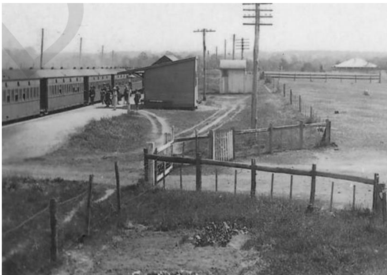
Figure 3.1 Doonside Railway Station in 1926, showing the original station building
