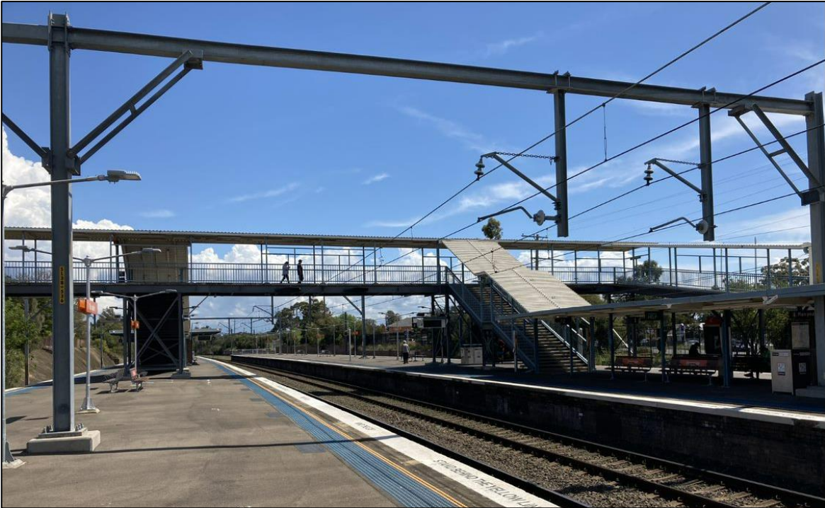
Photo 4.6 Doonside Station looking west to the Footbridge from the east end of Platforms 3 and 4
