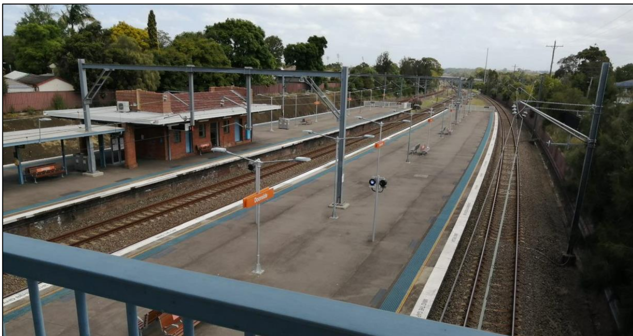
Photo 4.4 Views west from the Footbridge over the platforms to Station Building A
