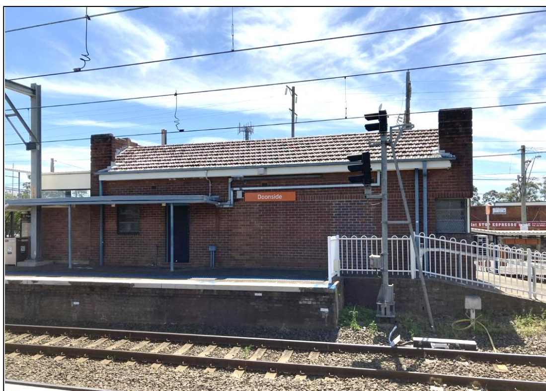
Photo 4.7 Station Building C showing the south elevation as viewed from Platforms 3 and 4
