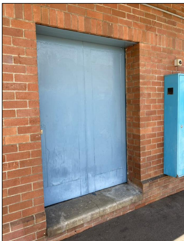
Photo 4.15 Station Building A, showing the original timber sliding door to the storeroom
