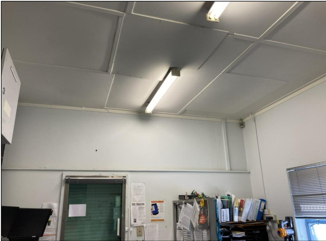
Photo 4.12 West end of Station Building C
