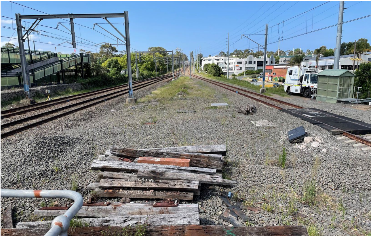
Photograph 4.9 Laydown area at the end of Platform 1 and 2
