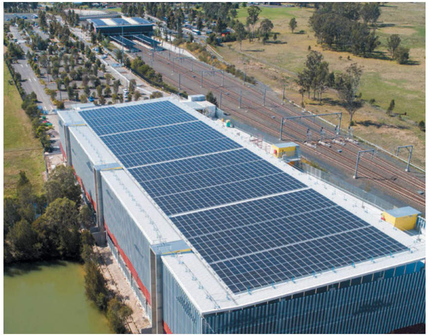
The rooftop has over 1300 solar panels to power the car park
