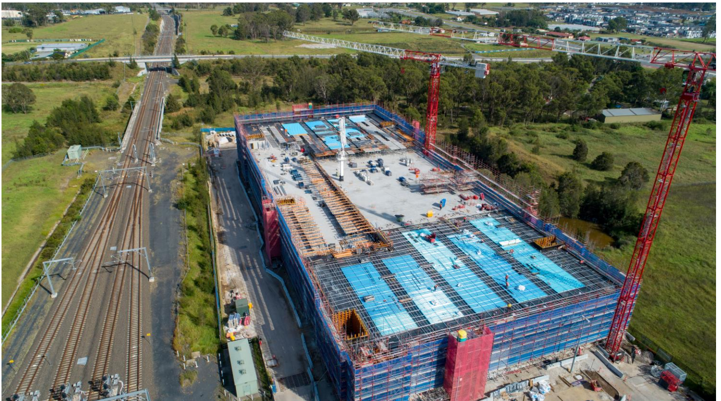
Construction progress on the new multi-storey car park at Leppington, March 2021
