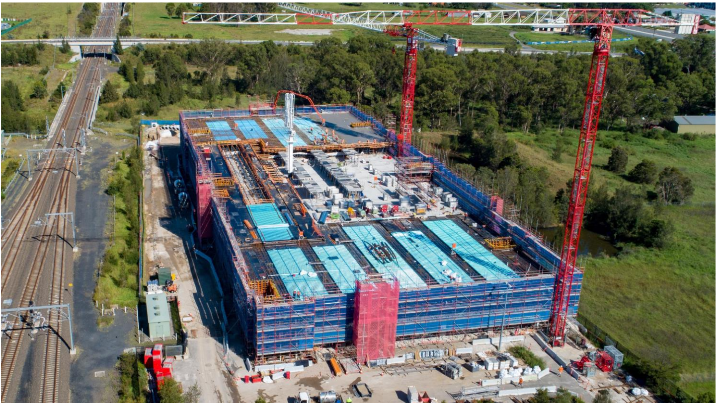
Construction progress on the new multi-storey car park at Leppington, February 2021
