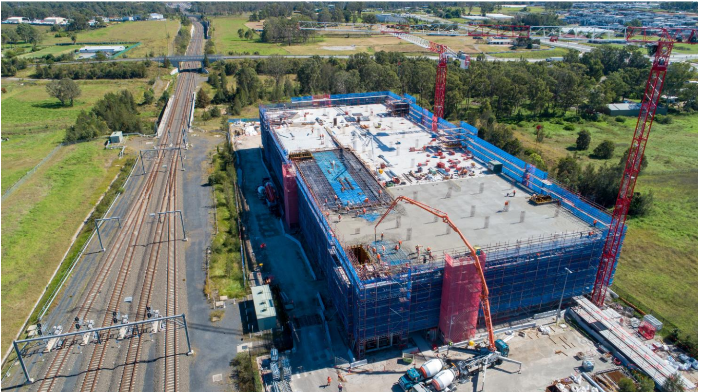
Construction progress on the new multi-storey car park at Leppington, April 2021
