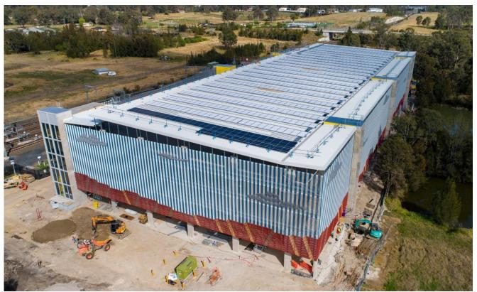
Construction progress on the multi-storey commuter car park at Leppington. In this photo you can see the solar panels being installed on the roof, one of the great sustainable features of the car park.
