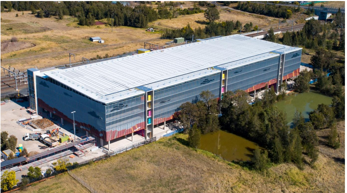
Progress photo of the new multi-storey commuter car park at Leppington.
