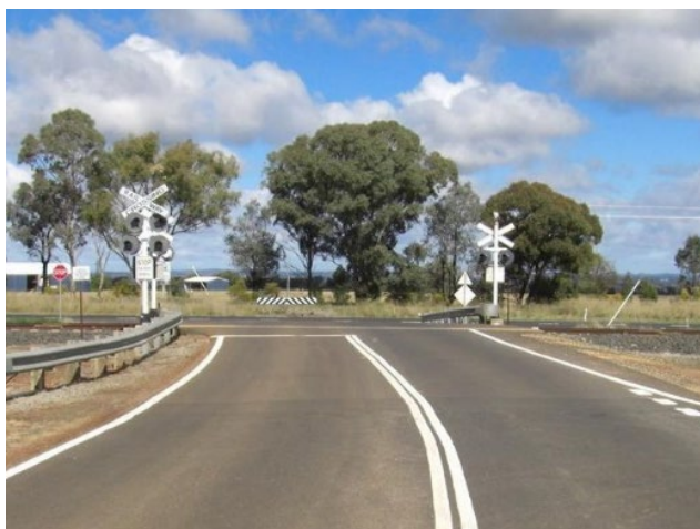
Figure 16: LX707 Eulomogo Road Dubbo (before and after)
