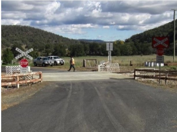
Figure 14: LX651 Tarana Road Tarana (before and after)
