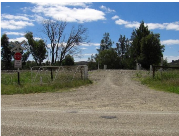
Figure 7: LX583 Jerrawa Road Jerrawa (before and after)
