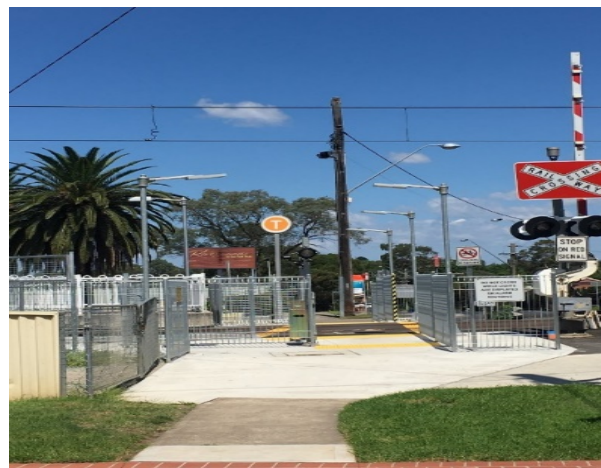
Figure 27: LX56 Bourke Street East Richmond – new country-side pedestrian swing gate crossing (left) and upgraded Sydney-side pedestrian crossing (right)
