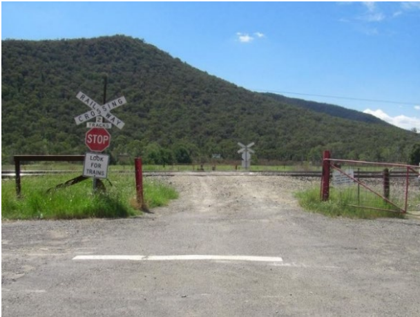
Figure 6: LX1908 Murrays Flat Road Towrang (before and after)
