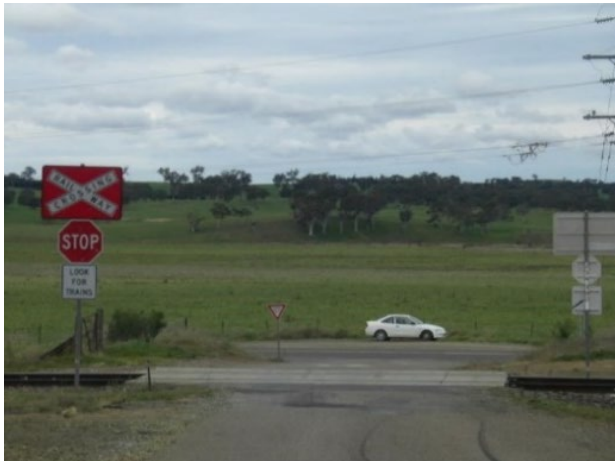
Figure 10: LX364 Covan Creek Road Lake Bathurst (before and after)
