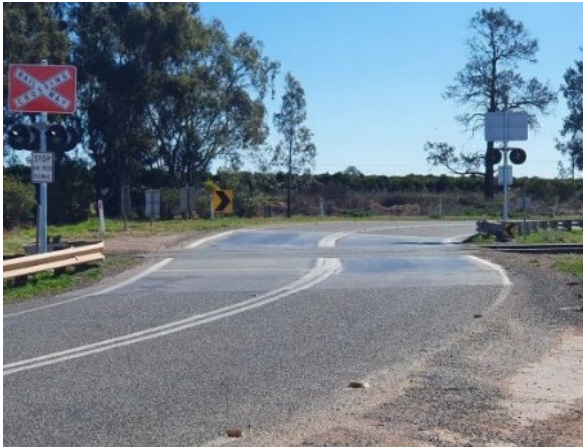
Figure 17: LX398 Irrigation Way Leeton (after)
