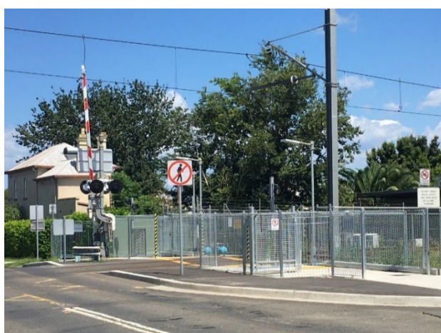
Figure 27: LX56 Bourke Street East Richmond – new country-side pedestrian swing gate crossing (left) and upgraded Sydney-side pedestrian crossing (right)
