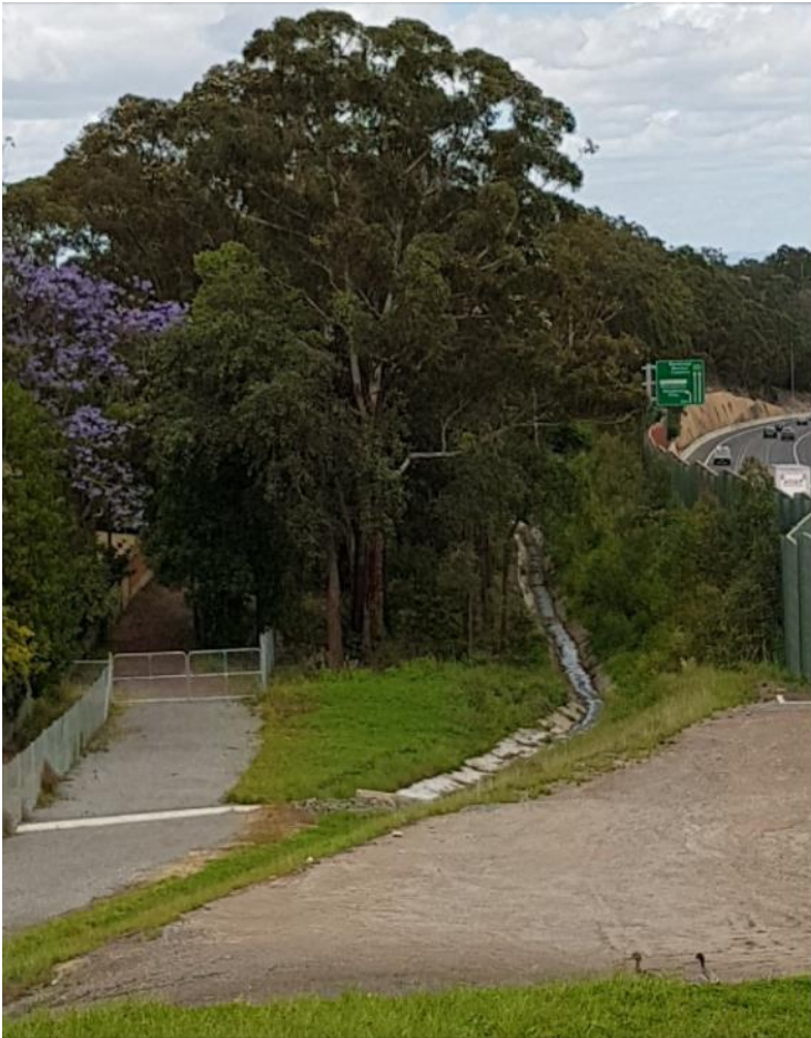
Figure 6-16 View downhill from the material stockpile toward the culvert-drain system with runoff toward Darling Mills Creek riparian corridor bushland (Source, Cardno, 2020).
