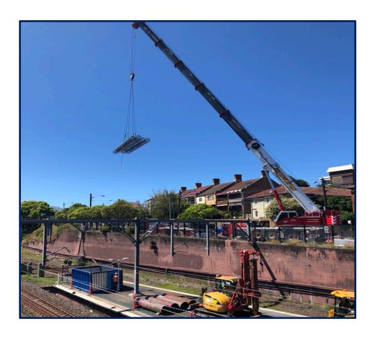
Above: crane on Trafalgar street lifting materials to prepare for the construction of the lift connecting the footbridge with platforms.
