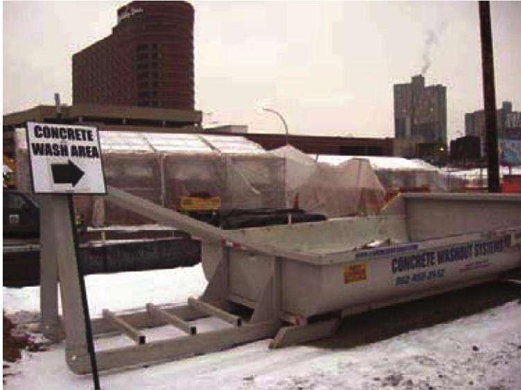
A skip washout system is capable of holding liquid and solid concrete washout materials until final treatment and disposal. Prevent commingling of other solid wastes with concrete washout materials.
