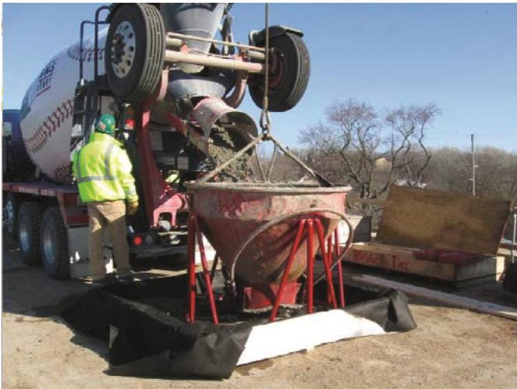
A rinse bucket separates concrete aggregate from washout water, and needs to be cleared of waste each day.
