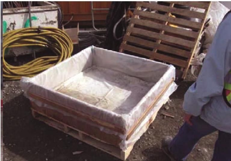
A sealed container that fits on a pallet for ease of removal can be used for small volumes. One benefit of this method is ease of moving the washout area to locations where concrete is being used. Do not completely fill the container, and beware of spillages when moving the pallet.
