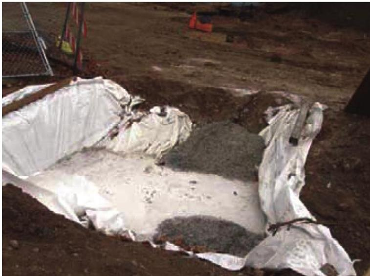
A lined trap system is excavated in an area with storm water overflow protection consisting of impervious plastic sheeting. The goal is to retain the liquids.
