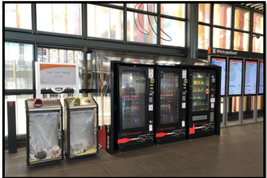
New SMART BIN technology installed behind the bins at the Gibbons Street entrance to Redfern Station.
