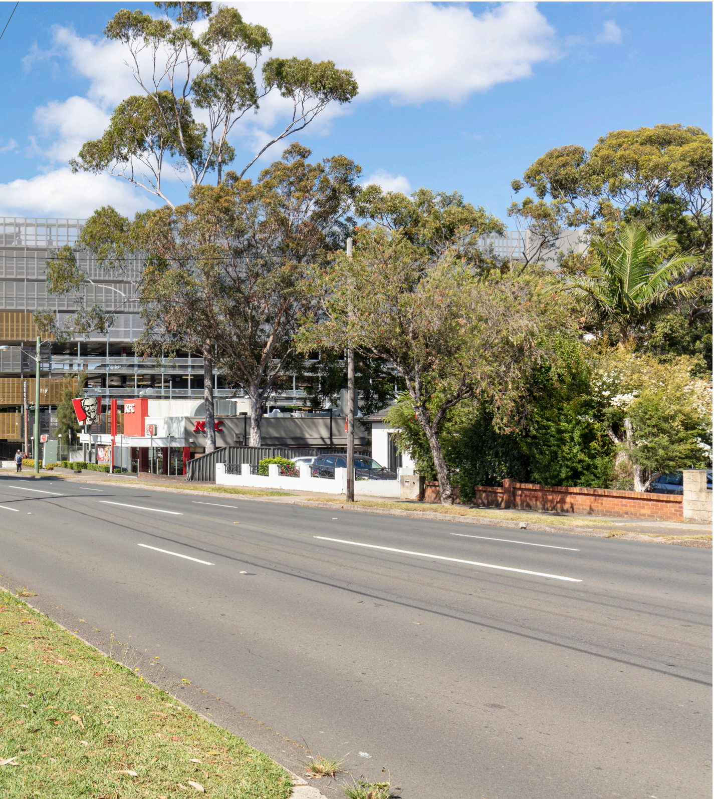
*Massing model shows the bulk and scale of the proposed MSCP expansion. Facade type and colouring will match the facade on The River Road frontage (as shown in Photomontage 1).
