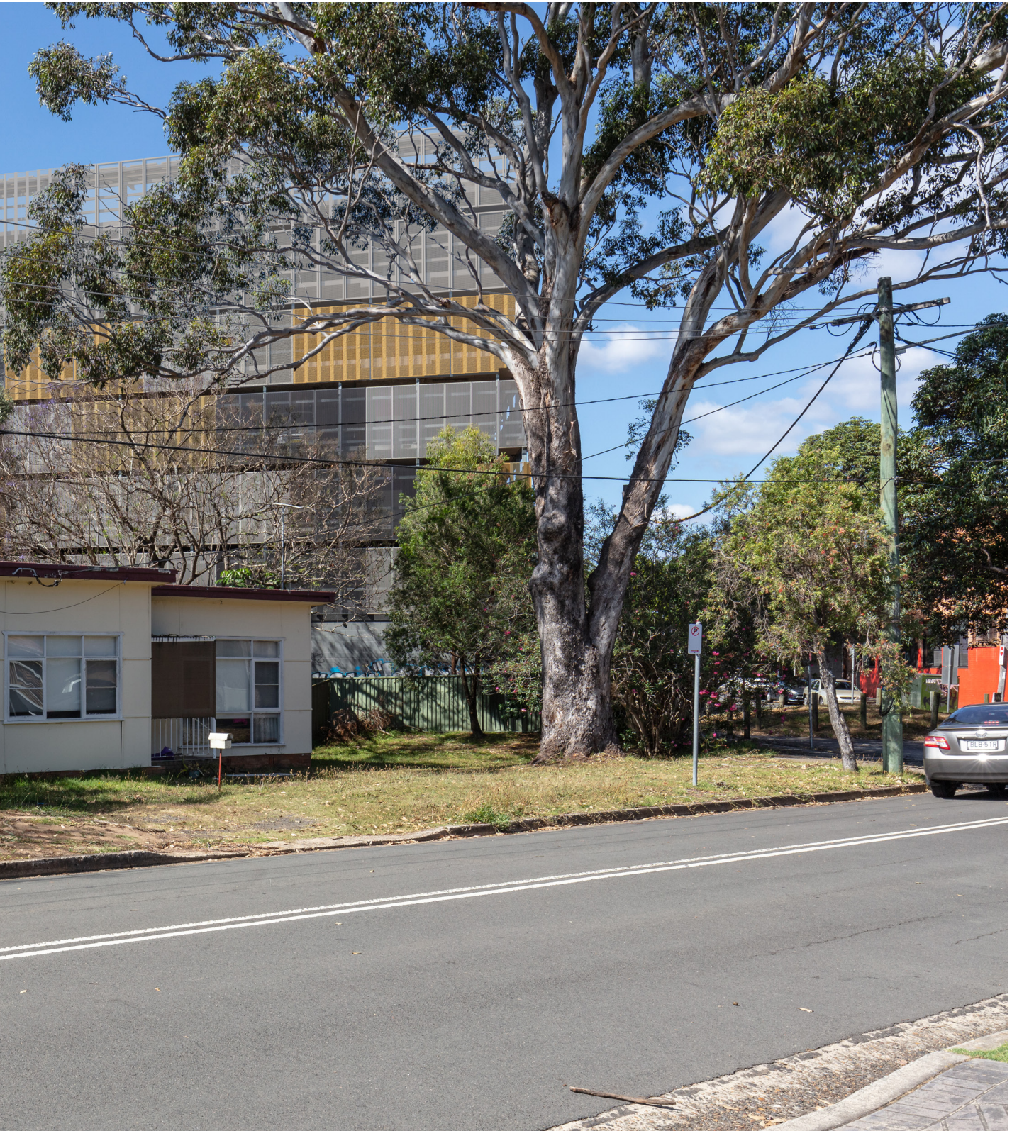
*Massing model shows the bulk and scale of the proposed MSCP expansion. Facade type and colouring will match the facade on The River Road frontage (as shown in Photomontage 1).
