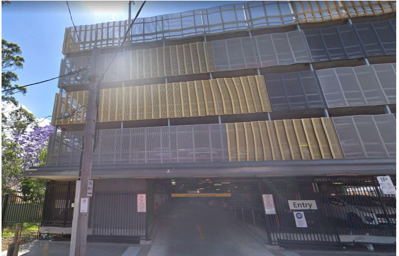
Figure 8 MSCP Simmons Street Entrance
