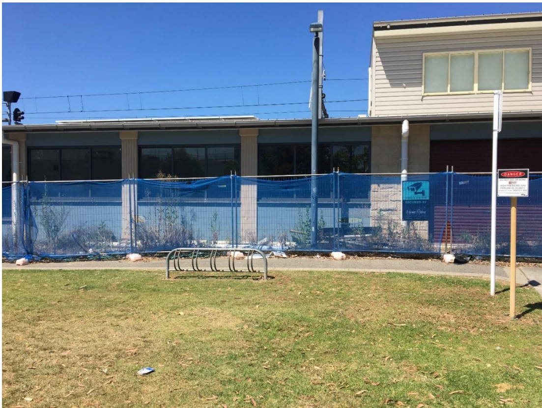
Figure 1-6 The existing bicycle rack at Revesby Station, proposed to be replaced, looking south
