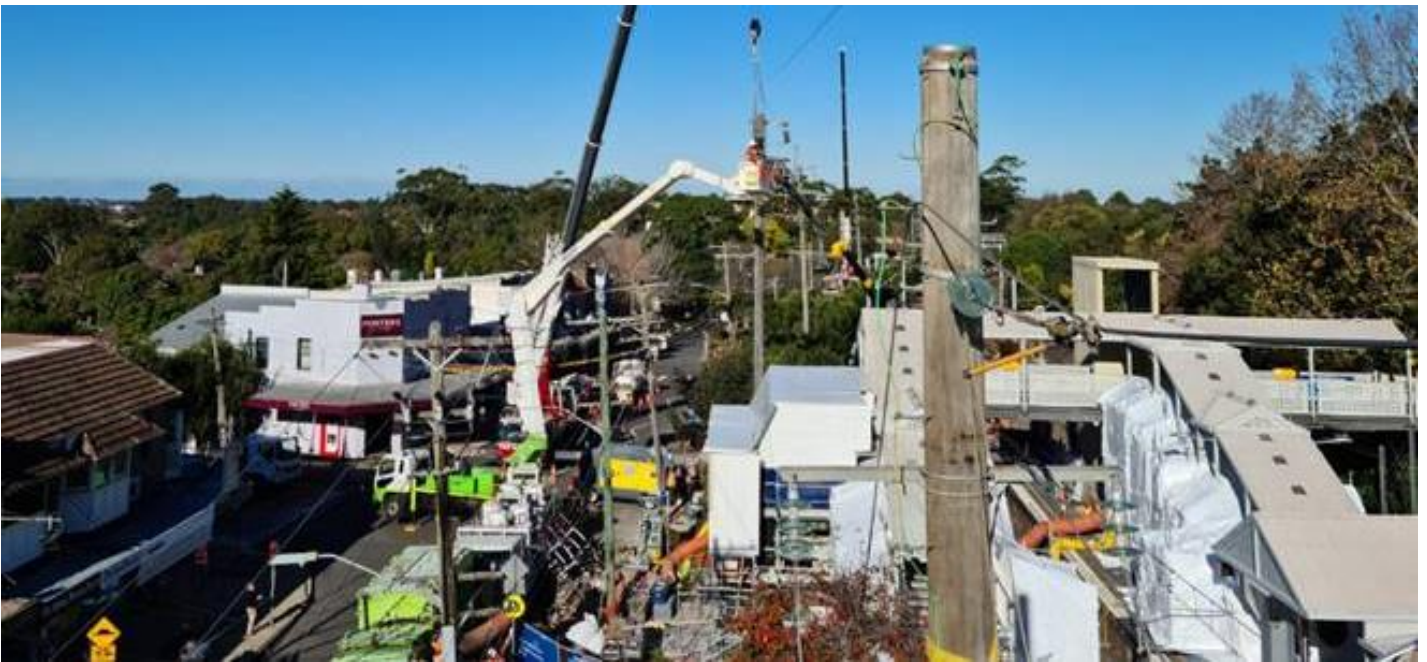
Aerial view of work being completed at Roseville Station during June 2021
