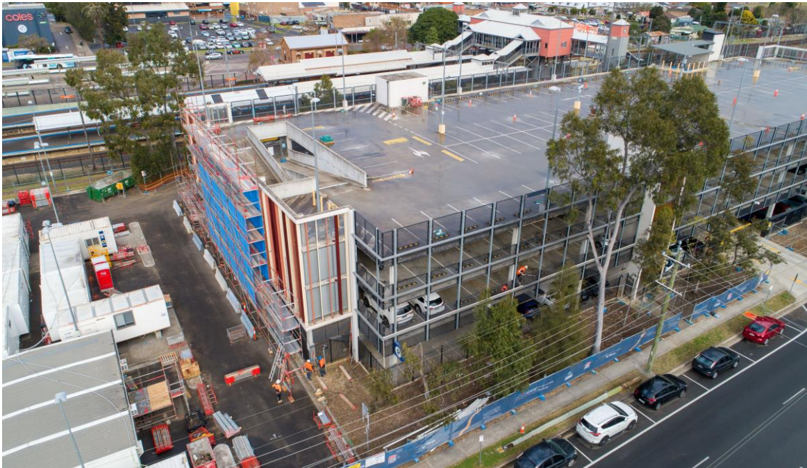
Construction progress on the new multi-storey car park at St Marys
