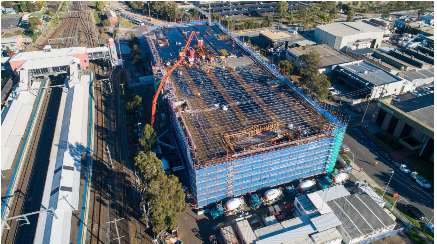
Construction progress on the multi-storey car park at St Marys
