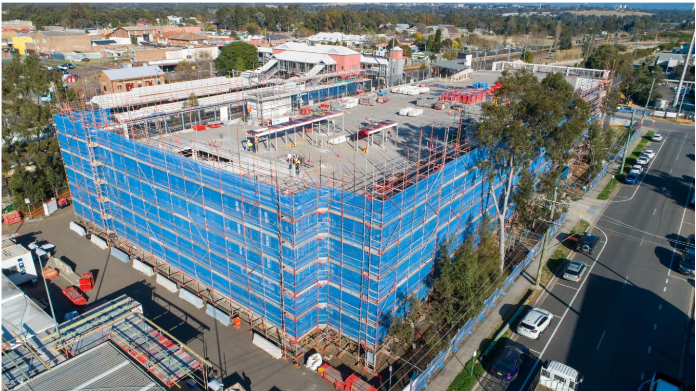
Figure 1 Construction progress on the new multi-storey car park at St Marys
