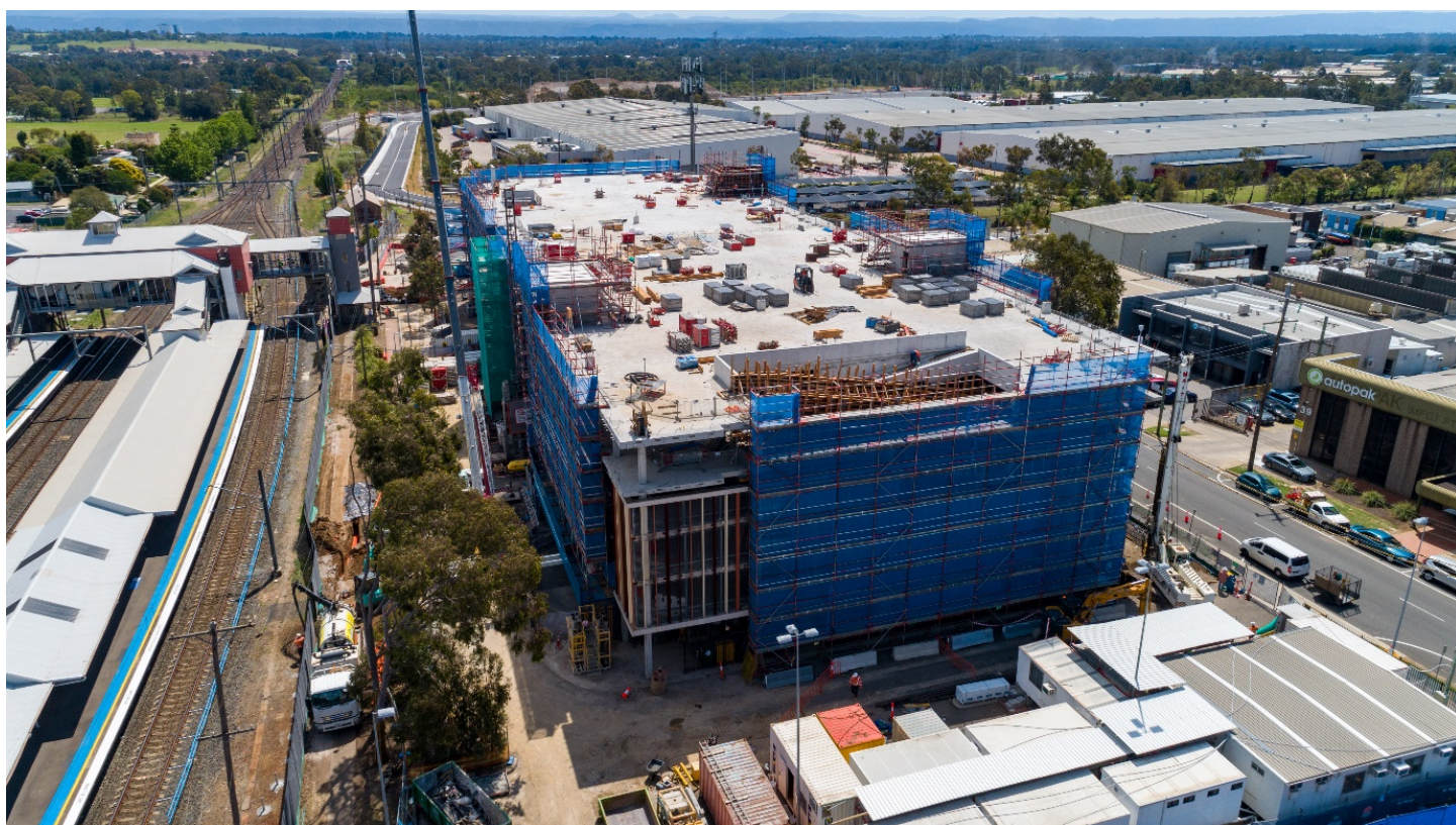
Construction progress on the multi-storey commuter car park at St Marys
