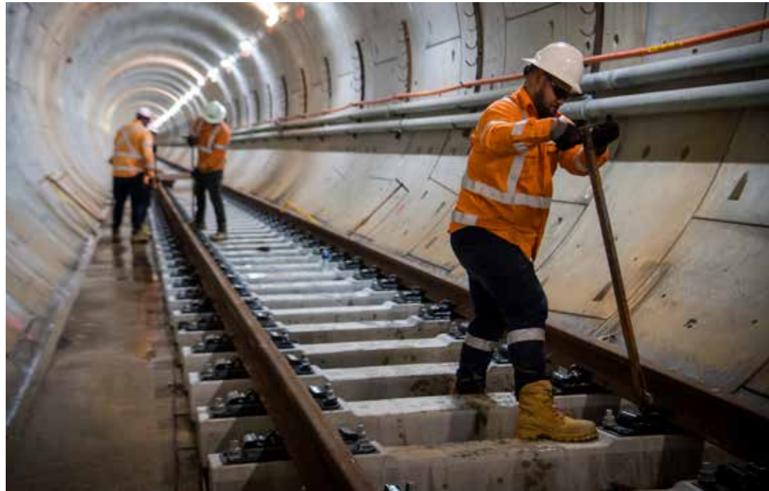
Concrete railway sleepers put in place and rail line assembled underneath Sydney Harbour.
