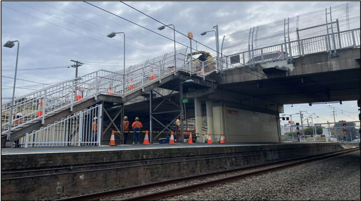
Figure 1-5 Photo showing the Reede Street overbridge and entry stairs to Turrella Station from the rail corridor
