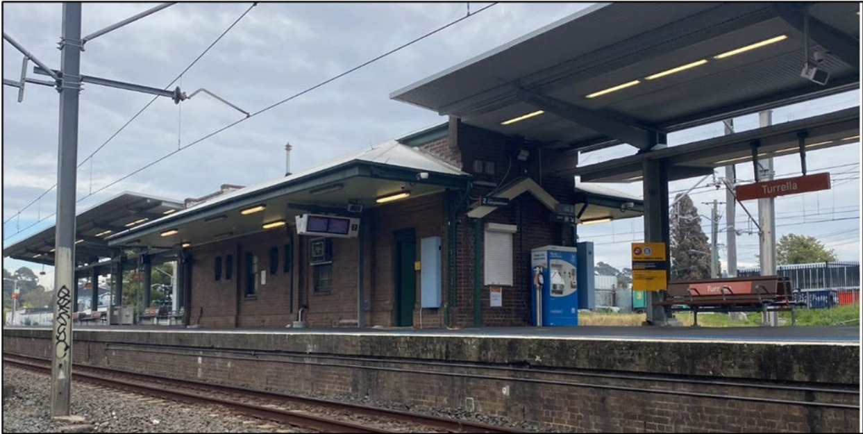
Figure 1-4 Photo showing Turrella Station platform and building, viewed from the south east from the rail corridor
