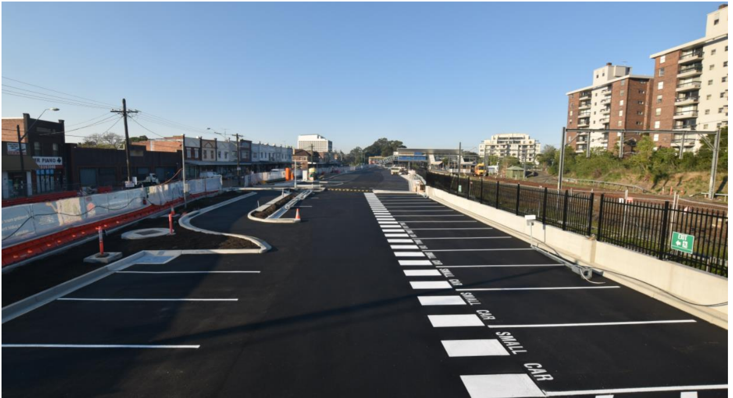
Construction progress on West Ryde Commuter Car Park, September 2021
