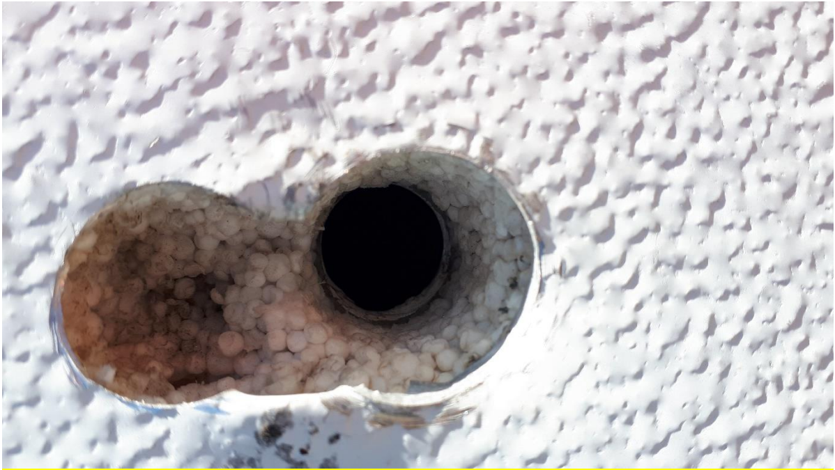
Photo 2 – Foam filled sheet metal panels from wall and roof
