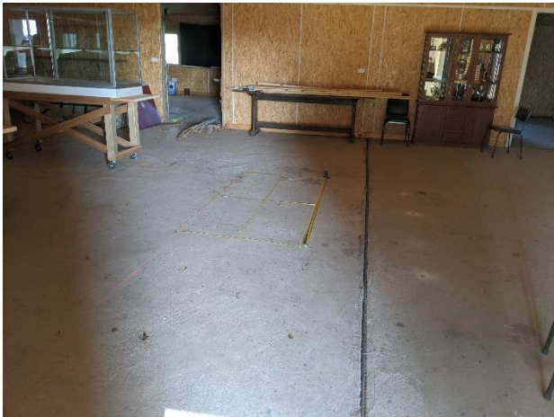
Photo 27 Tarago Showground, interior of building. Date: 26/03/20
