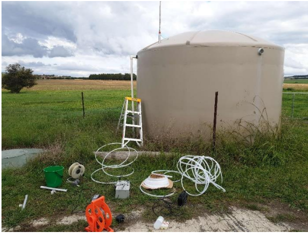
Photo 25 Water tank at the Tarago RFS. Date: 25/03/20
