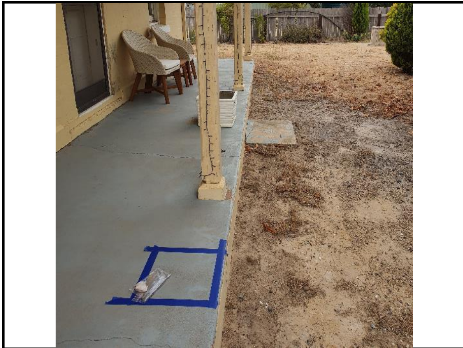
Photo 12: Station Masters Cottage external dust sample location (SWAB17) facing west. Taken 19/12/19.
