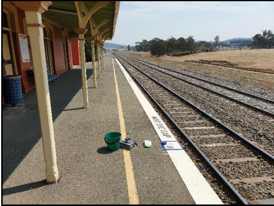
Photo 5: Tarago Station platform facing south. Taken 19/12/19.
