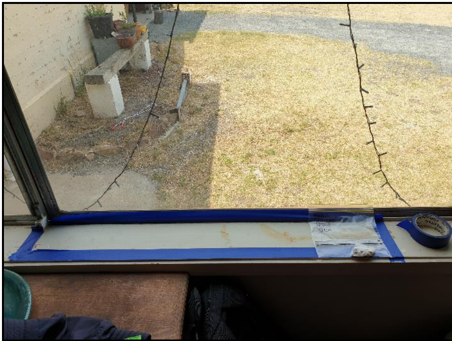
Photo 14: Station Masters Cottage internal dust sample location (SWAB19). Taken 19/12/19.
