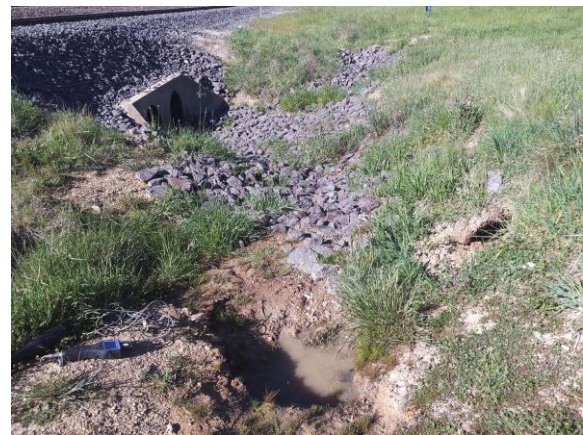
Photograph 6: Location of SW5 / SED5. Sampled 13 October 2020. Water not flowing.
