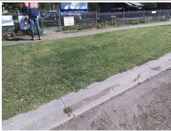
Photograph 17: Location of XBRAID003, XRF measurement of sediment within drainage line west side of Braidwood Road, adjacent school. No water present.
