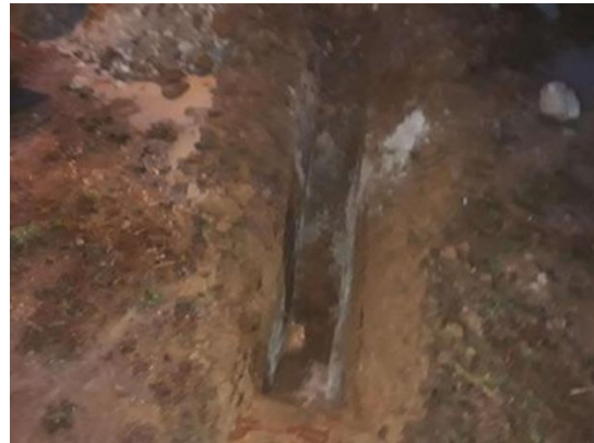
Photograph 36: Test pit LO_TP06 terminated at 1.5 mbgl.
