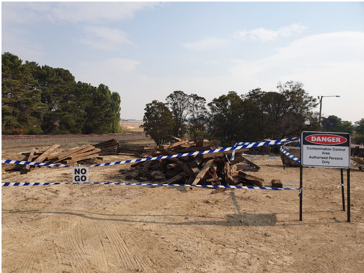
Photo 1 – Location of sleeper within the rail corridor
