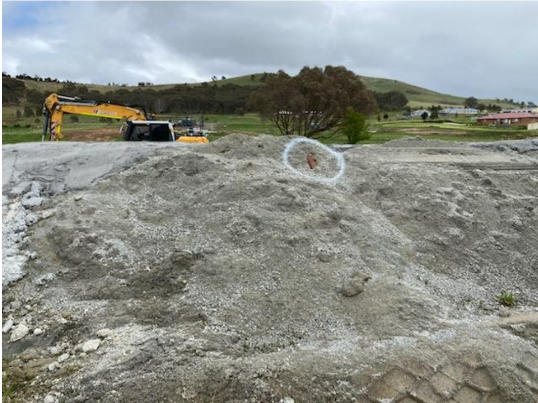
Central Eastern Face – Prior to final application of capping
