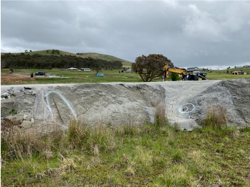
South Eastern Face – Prior to final application of capping
