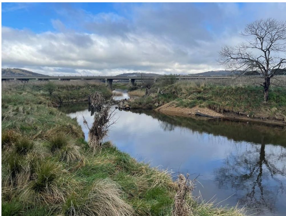
Photo 8: Sample location SW9 within Mulwaree River adjacent to Braidwood Road, facing west (13 September 2022)
