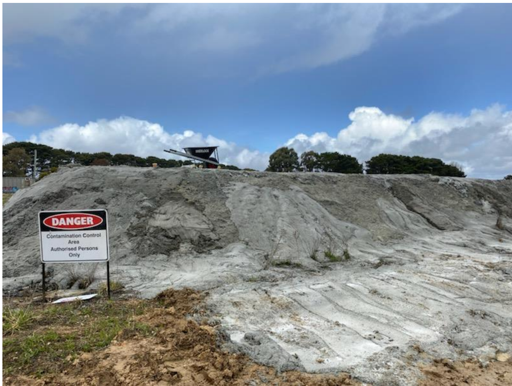
North Western Corner – Post final application of capping
