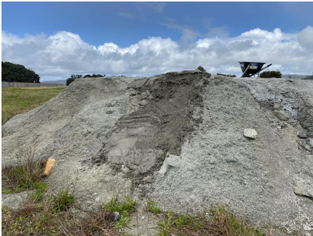
North End – Post final application of capping
