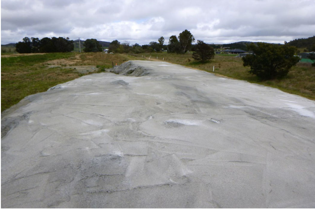
Photo 3: Stabilised sand applied as stockpile capping (top of stockpile)
