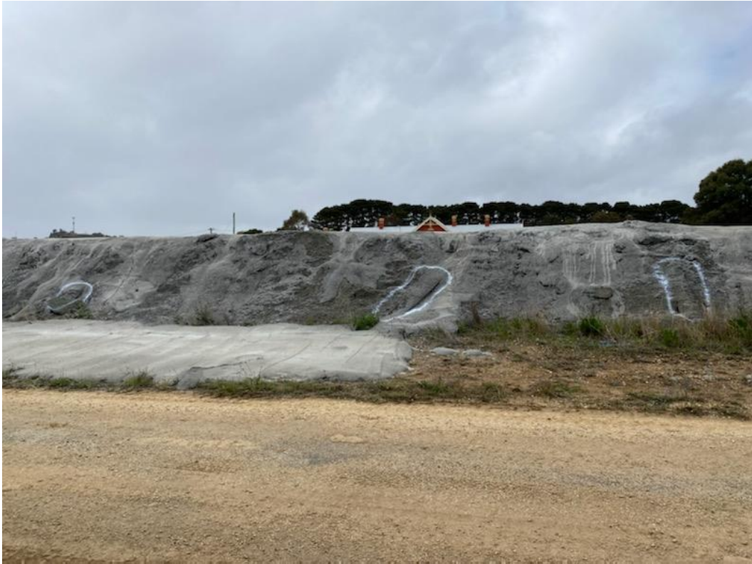
North Western Face – Prior to final application of capping
