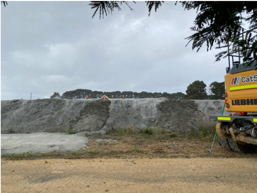
North Western Face – Post final application of capping
