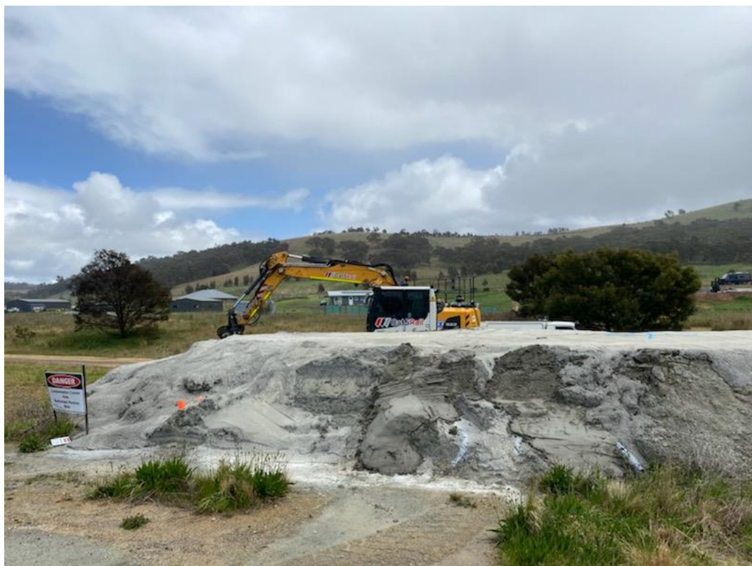
South Eastern Corner – Post final application of capping
