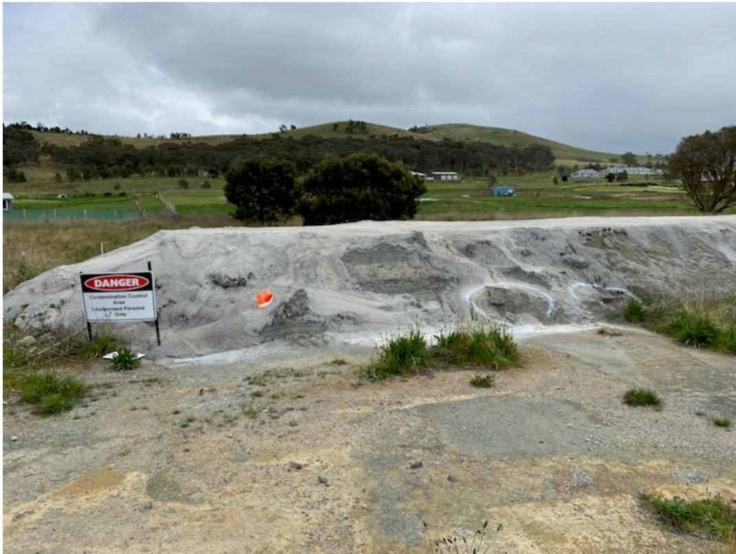
South Eastern Corner – Prior to final application of capping
