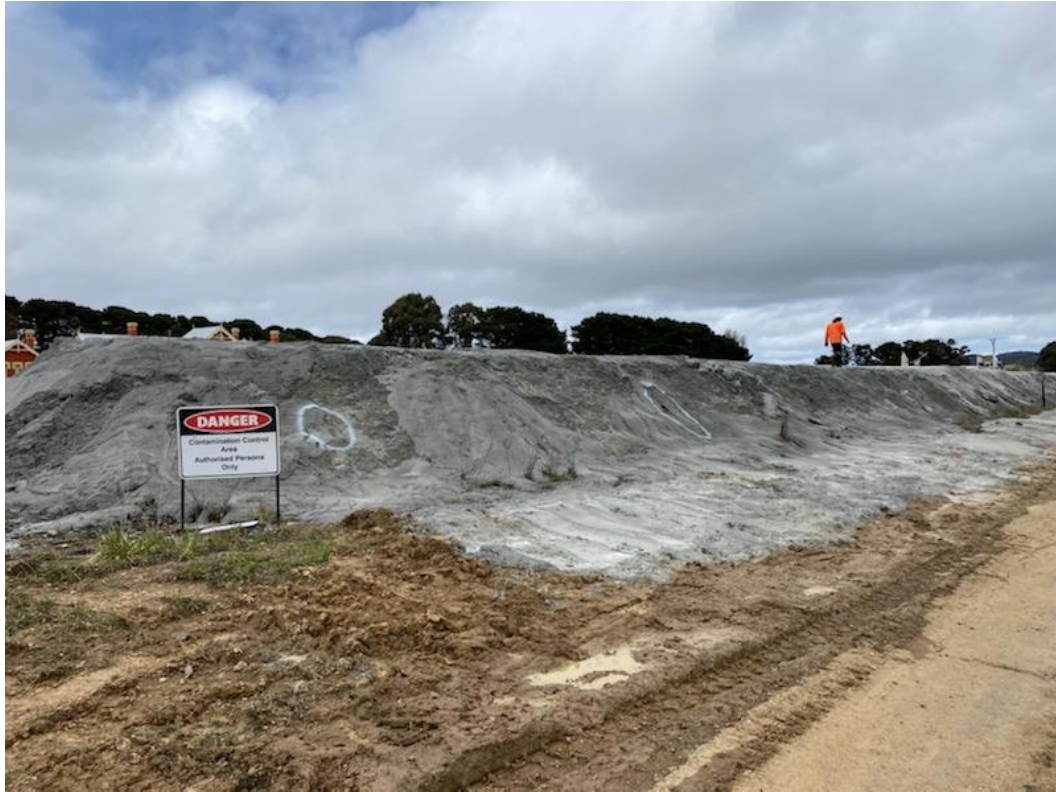
North Western Corner – Prior to final application of capping
