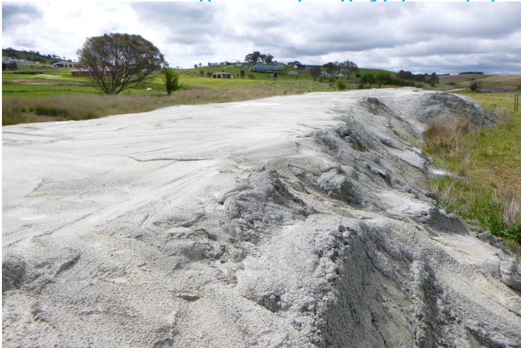
Photo 4: Stabilised sand applied as stockpile capping (top and eastern side of stockpile)
