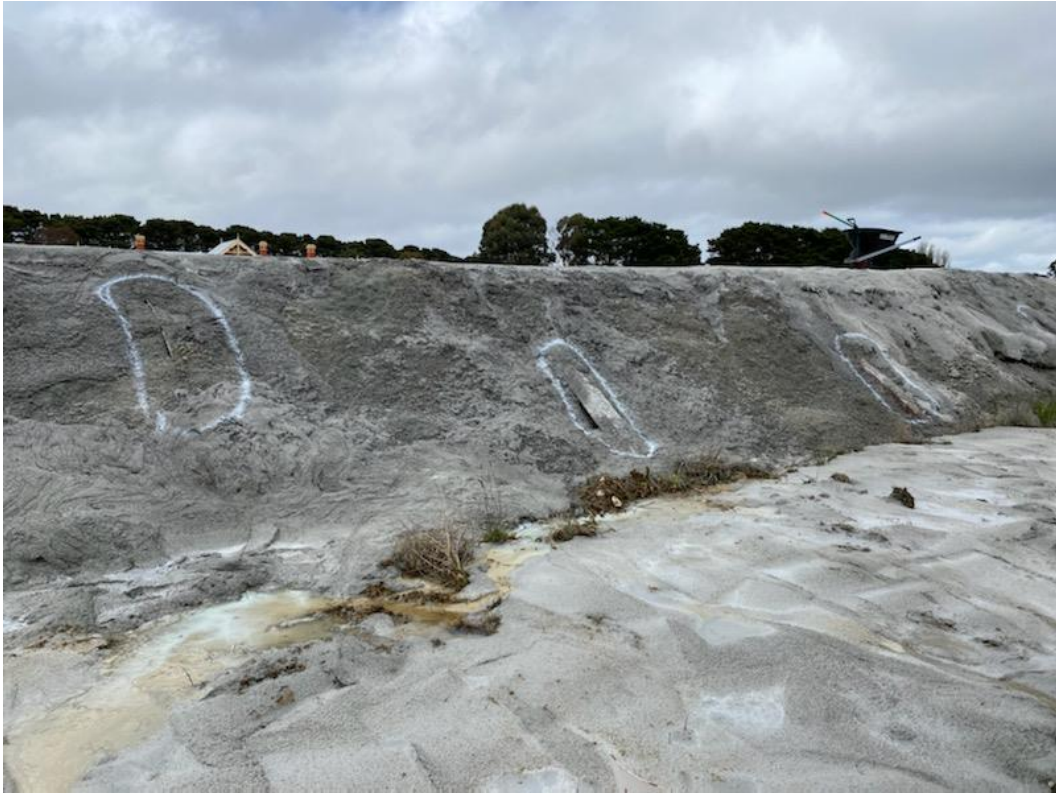
Central Western Face – Prior to final application of capping
