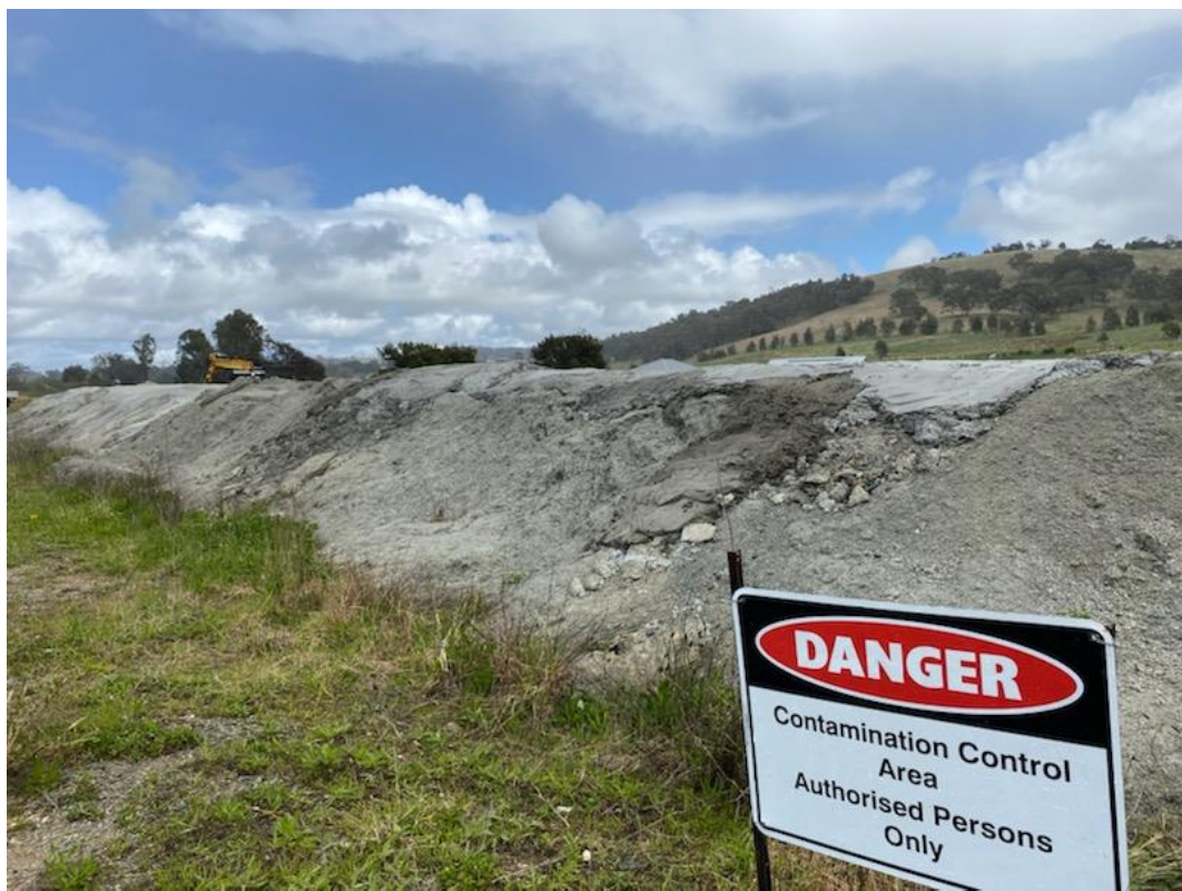
North Eastern Face – Post final application of capping
