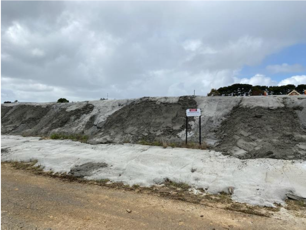
Central Western Face – Post final application of capping
