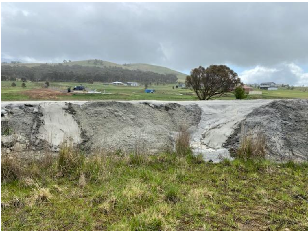
South Eastern Face – Post final application of capping
