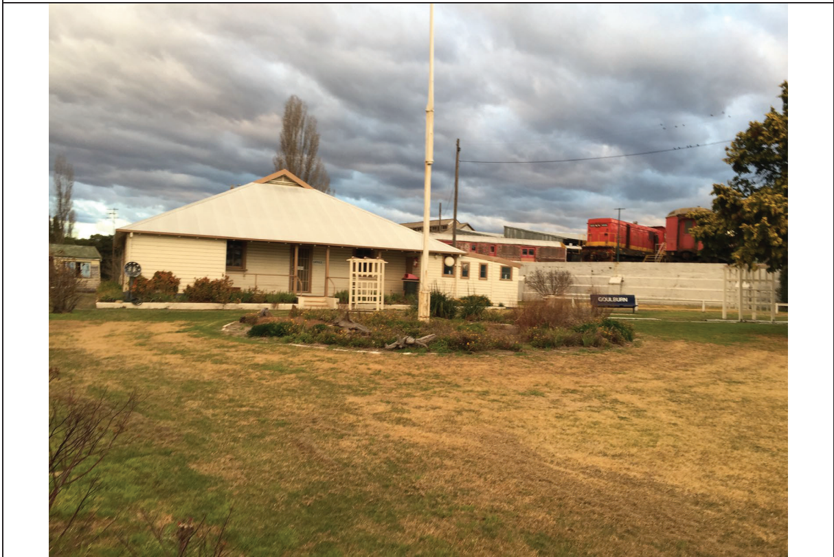
Photograph 2 View southwest towards the Administration Building, located to the east of the Roundhouse Building.
