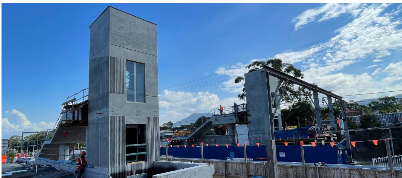
Pictured: All scaffolding has been removed from the lift shafts revealing the custom-made concrete panels.
