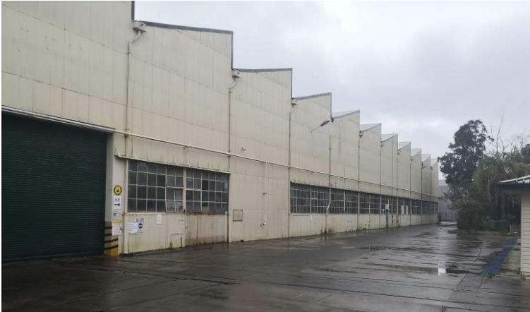
Figure 5 View of the South Elevation
