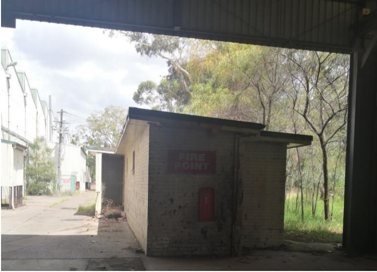
Figure 13 View of the second toilet block – to be retained subject to approval from the NSW Fire Brigade for the required access road
