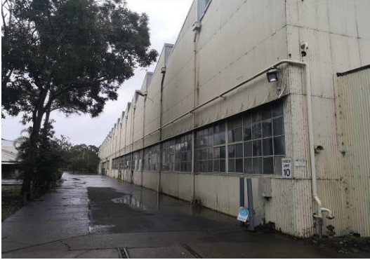
The South Elevation of the Tank Annex
