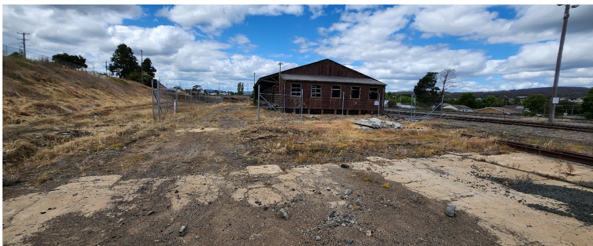
Plate 12. Timber and metal building (off site)
