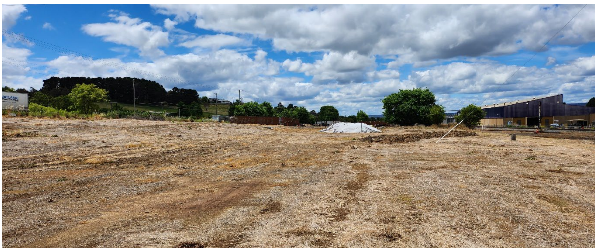
Plate 6. Wheat yard siding looking north, with covered material stockpile
