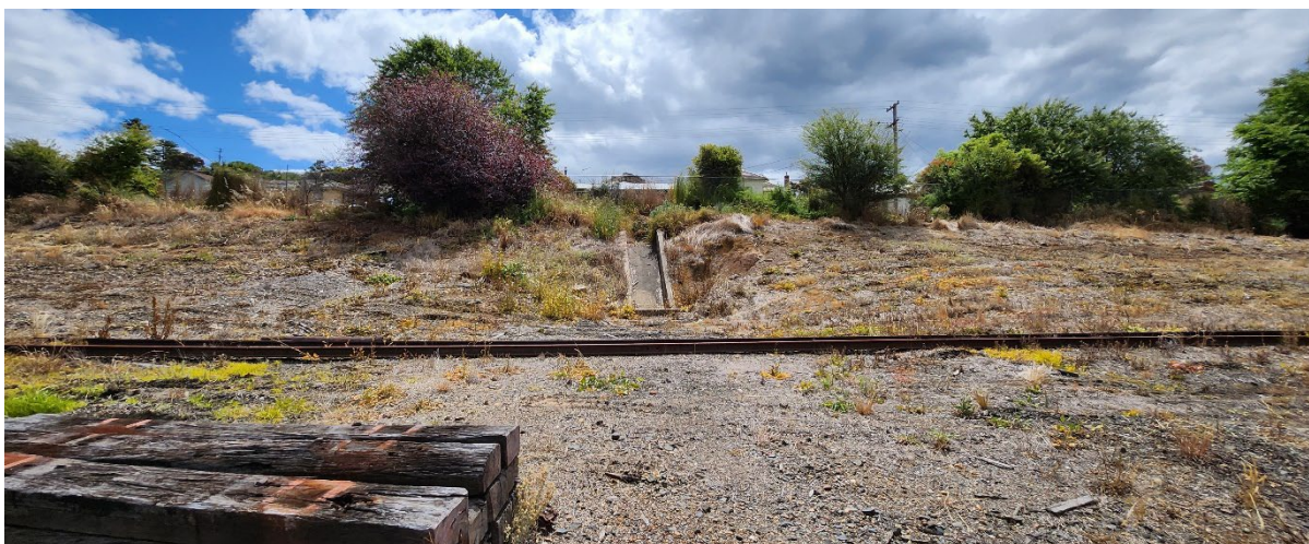
Plate 10. Stormwater infrastructure from Sloane Street
