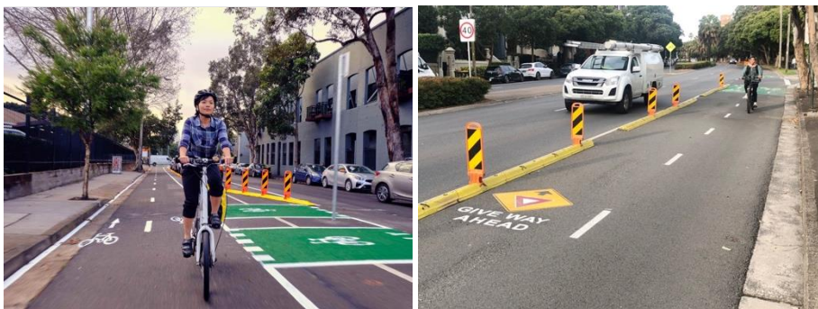
Figure 7. Left: Henderson Road pop-up cycleway at up to 3.5 metres. Image credit: City of Sydney. Right: Moore Park Road pop-up cycleway at 3 metres. Image credit: Mike Harris.
