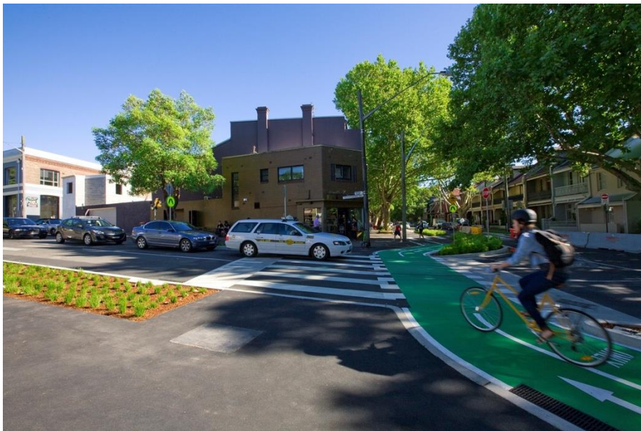
Figure 20: Bent-out crossing on Bourke Street Cycleway. Image credit: Group GSA/ Simon Wood.
