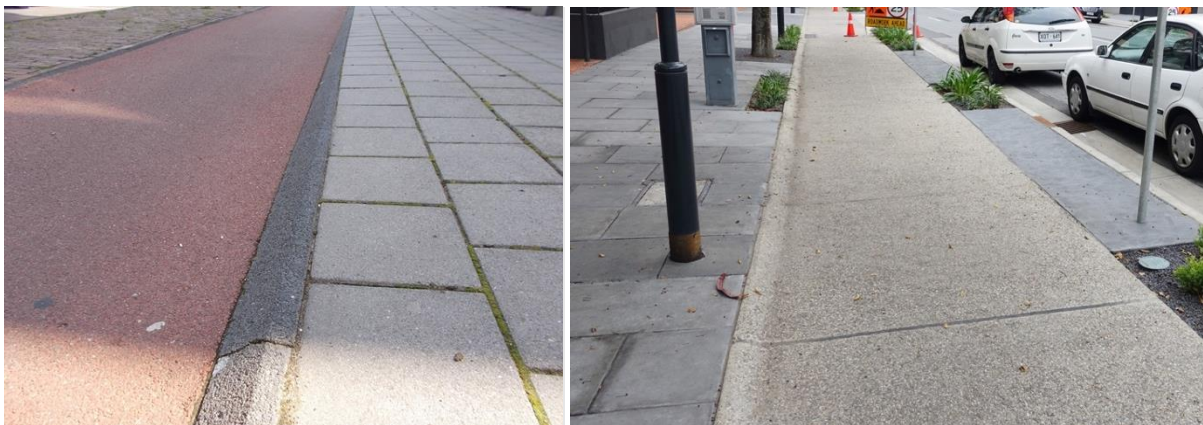
Figure 9: Left: A stepped kerb cycleway with a precast mountable kerb to the footpath in the Netherlands. Image credit: Mark Philpotts. Right: A stepped kerb cycleway with an in-situ mountable kerb to the footpath in Adelaide. Image credit: Mike Harris.
