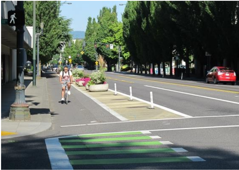
Figure 11. Retrofitted separated bicycle path in Portland, Oregon. Image credit: Monsere, Dill, McNeil, et al., (2014).
