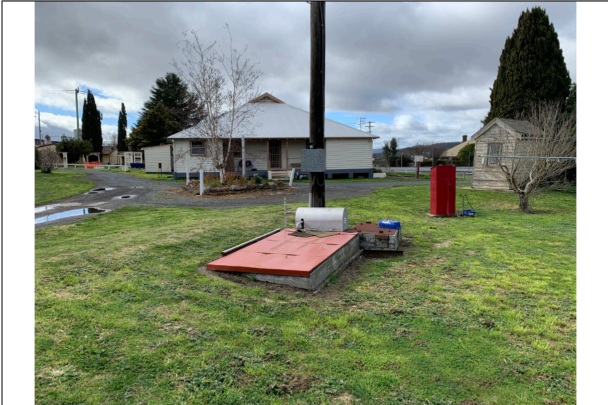
Photograph 17 View east towards the stormwater pit in the eastern portion of the site.
