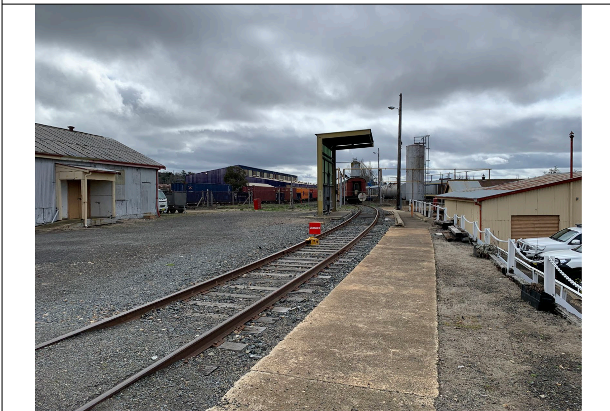
Photograph 6 View north towards the decommissioned refuelling gantry.
