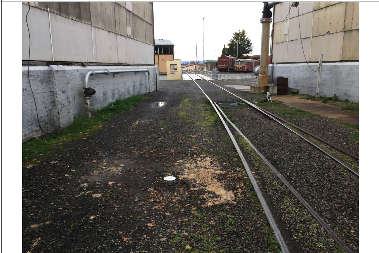
Photograph 18 View north towards groundwater monitoring well MW06 (foreground), and the turntable (background).
