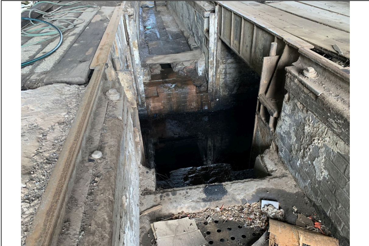
Photograph 9 Locomotive maintenance pit within the southern portion of the Roundhouse.
