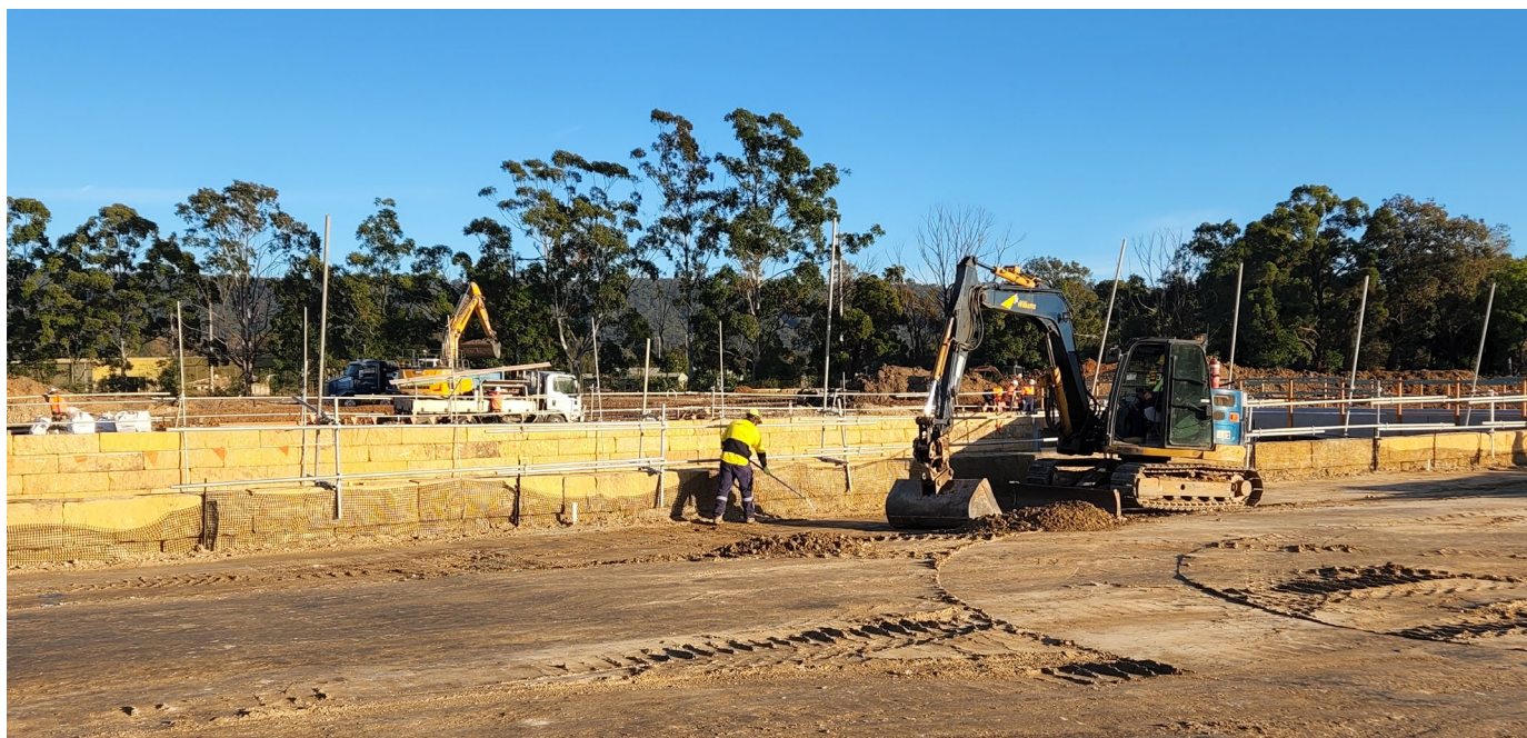
Work progressing at the new Emu Plains Commuter Car Park
