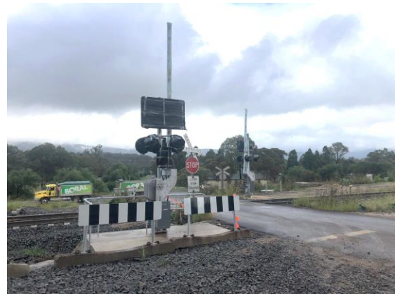
Figure 26: Gateleys Road after
