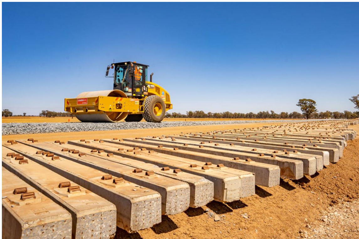
Figure 33: Development work on the Inland Rail project
