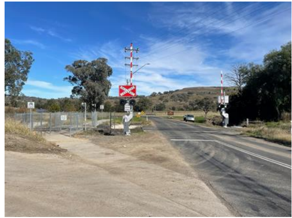
Figure 13: Merriwa Road after
