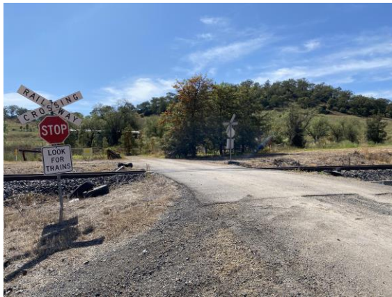
Figure 25: Gateleys Road before
