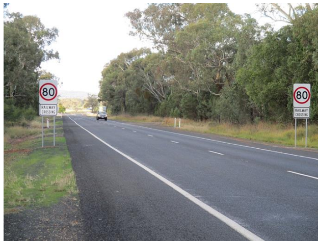
Figure 31: Golden Highway, Beni speed reduction from 100km/h to 80km/h
