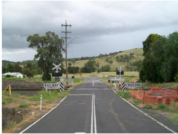
Figure 12: Merriwa Road before
